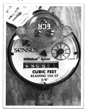
Some meters are newer models that have digital (LCD) display readouts with solid plastic lids. In this case, the lid must be opened to access the face. The reading will only be visible for a short time. It will shut off after a moment to preserve battery strength. If this happens, shut the lid securely, wait a moment and open it, and the reading should be visible once again. The numbers are read the in the same way, from left to right.
