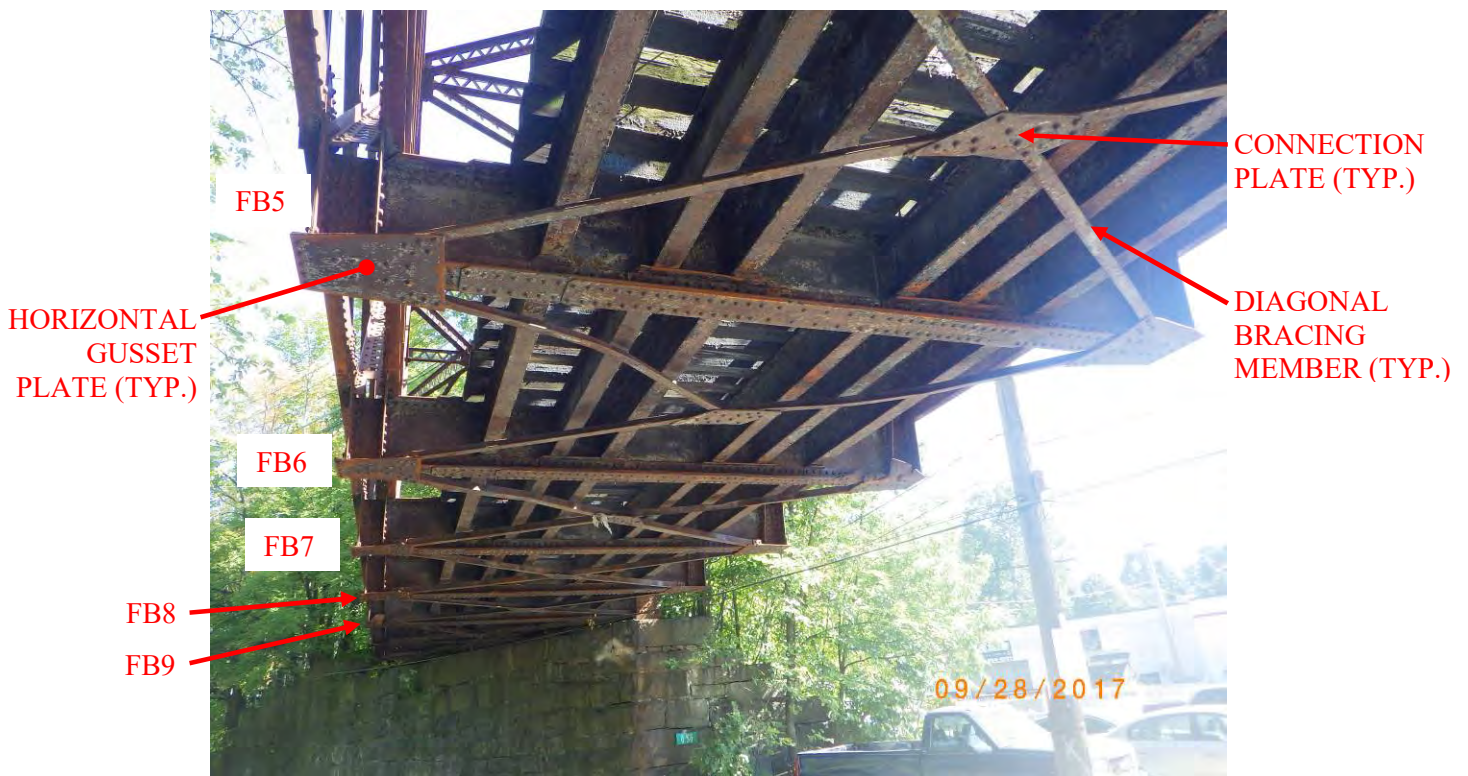
Photo 1: Overall underside view, looking east.
