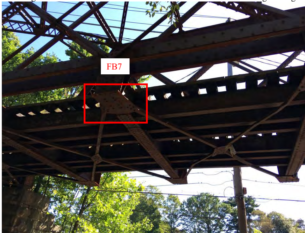
Photo 3: Floor beam 7, north side, looking south.
