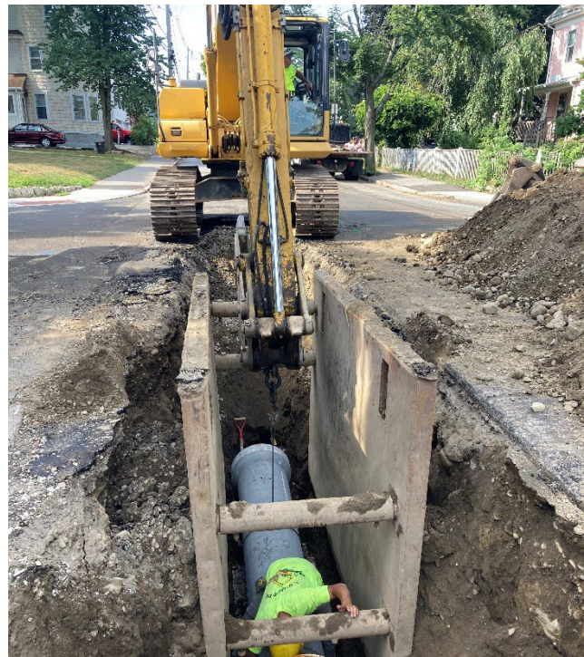
Stormdrain Replacement and Improvements – Ash and Lowell Streets – Completed in Year 2020
