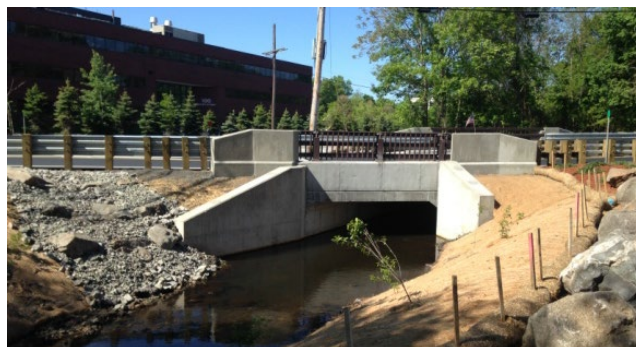
Culvert Replacement - Beaver Street
