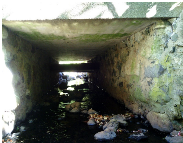
Culvert inspection – Stanley Road
