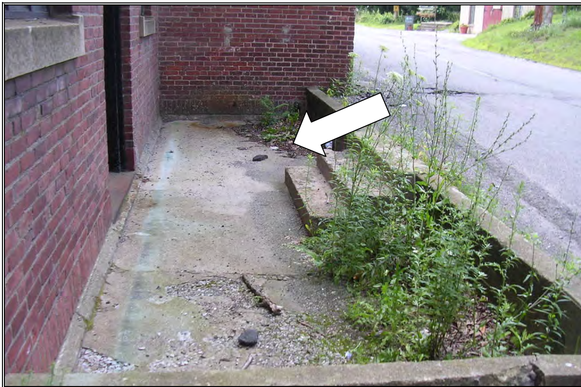
Photo Number 51: Former location of gasoline UST (formerly used for Power Plant generator)
