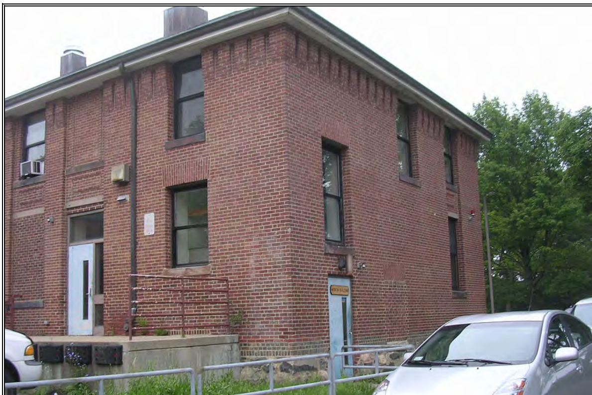
Photo Number 27: Northeast corner of North Building.
