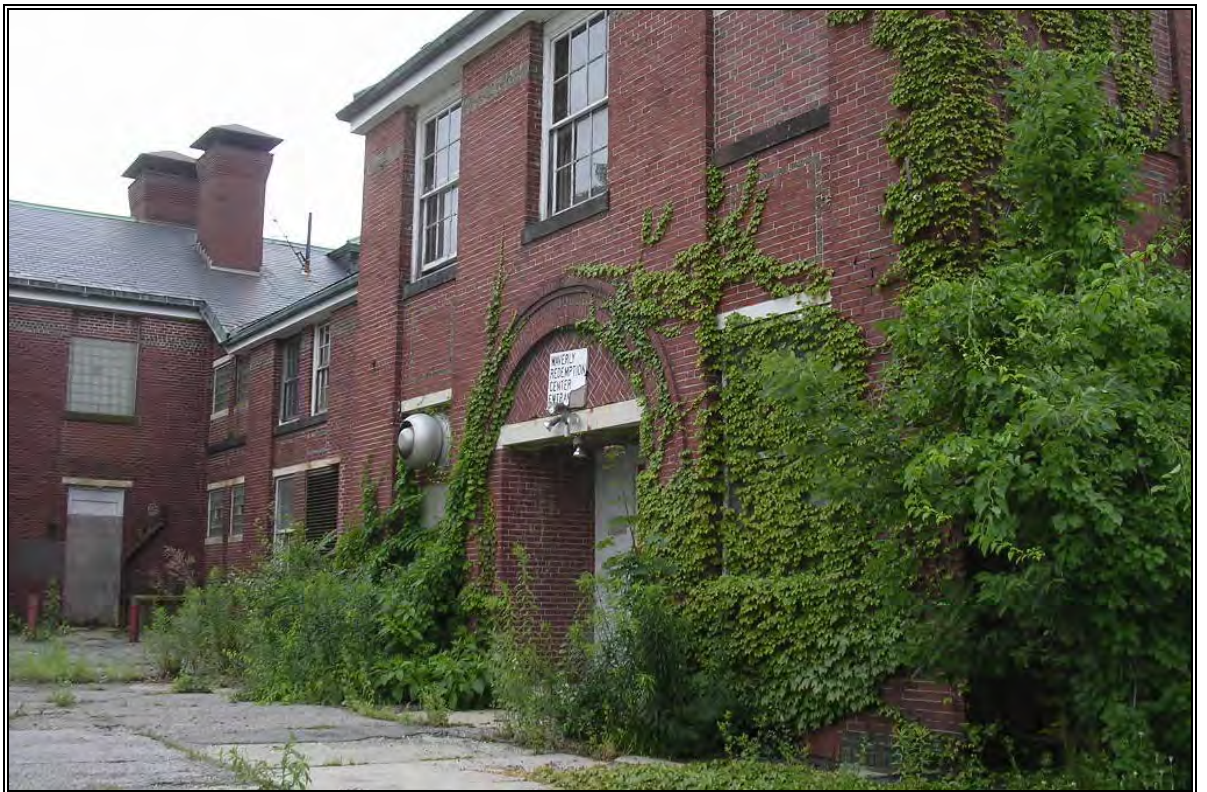
Photo Number 10: North side of East/Dowling Hall and parking lot impacted by gasoline release.
