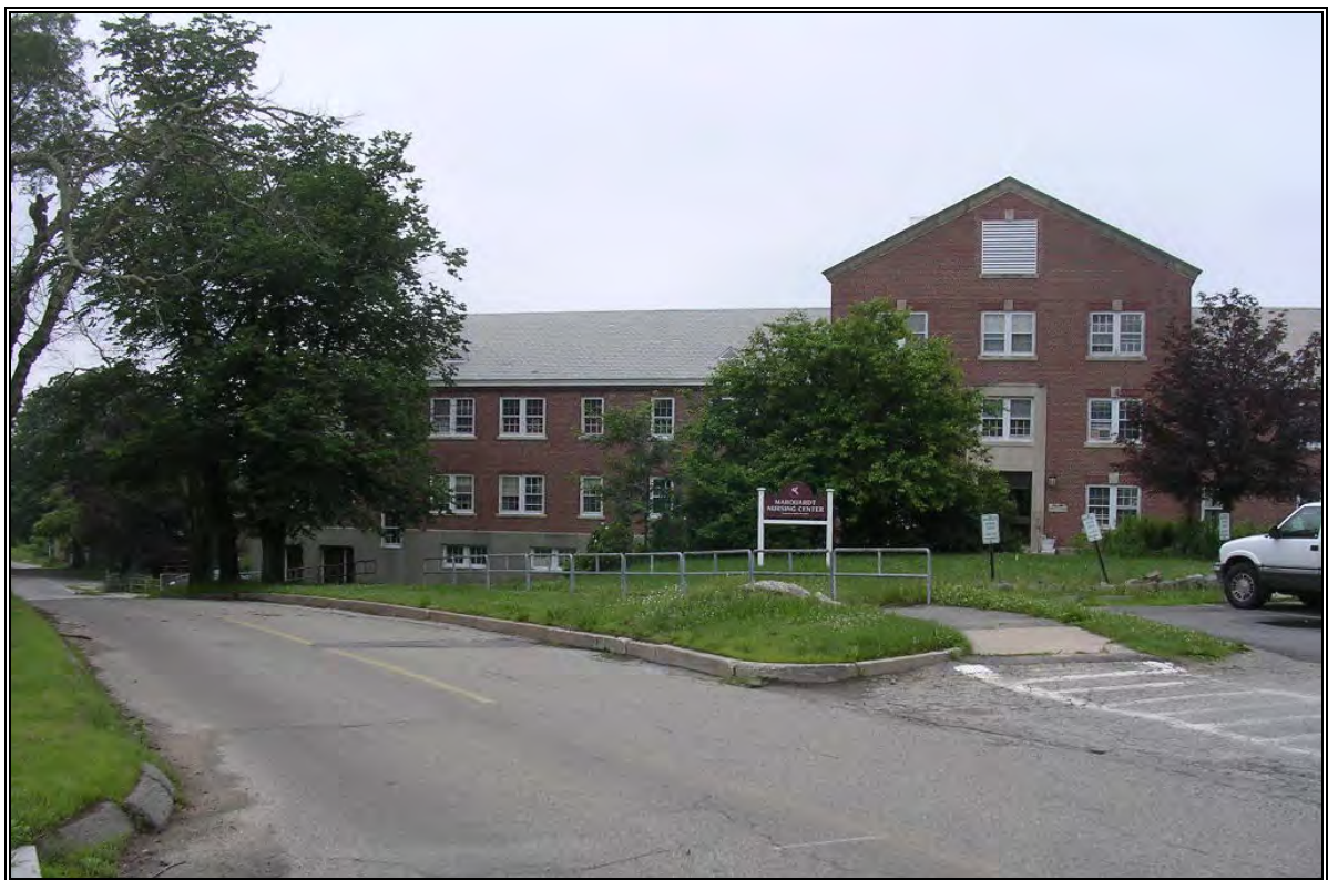
Photo Number 8: Northwest side of Thom Building occupied by the Marquardt Nursing Center.
