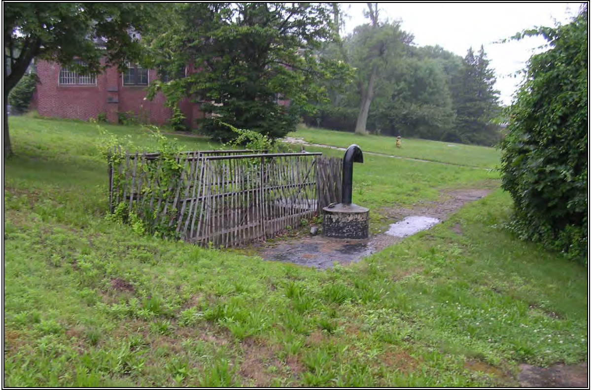
Photo Number 33: Access and vent pipe to steam pipe subway.
