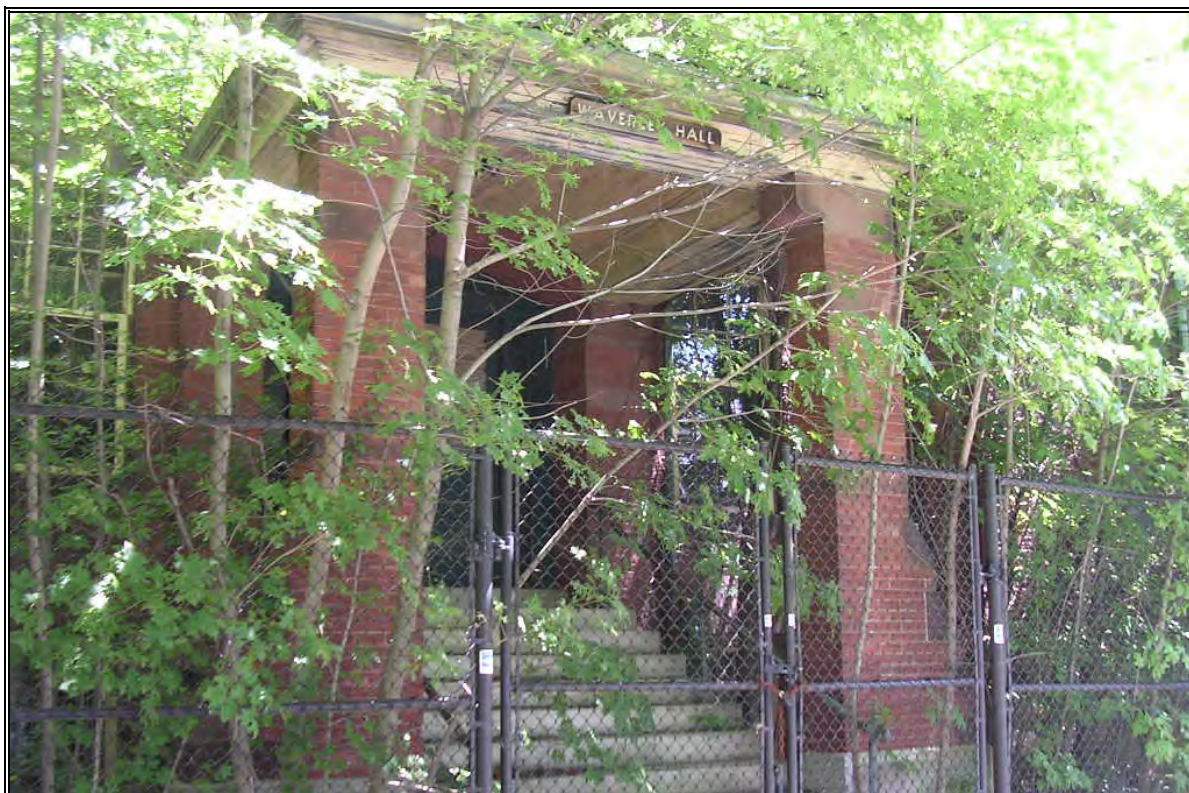
Photo Number 37: Waverley Hall entrance secured behind chain link fencing.
