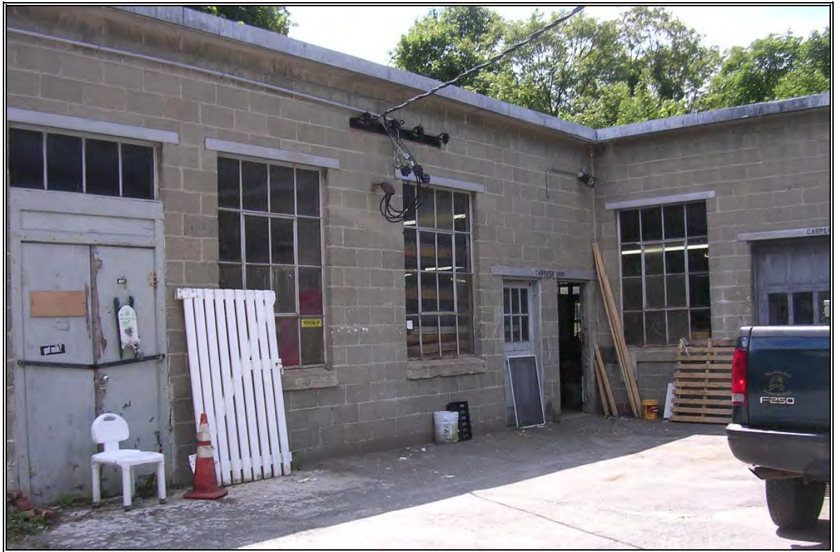
Photo Number 45: East side of Maintenance buildings and workshop entrances.
