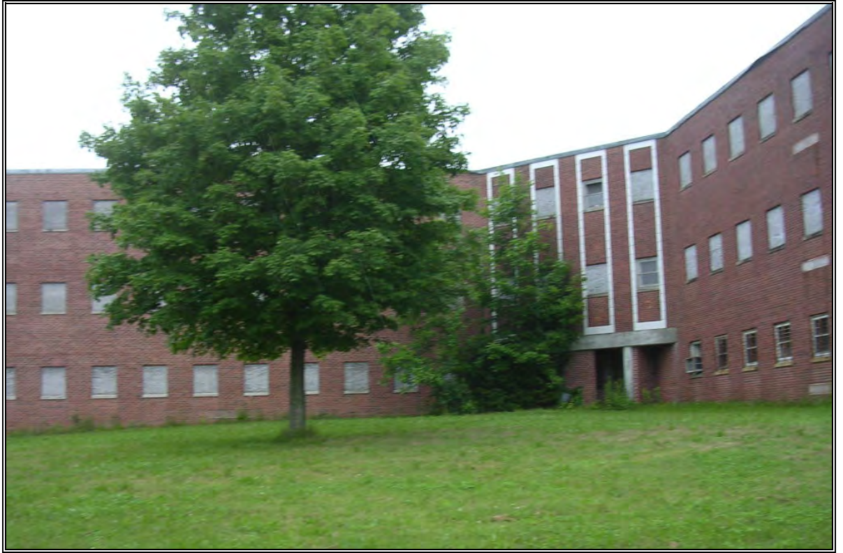
Photo Number 31: Northwest side of Kelley Hall which was boarded up.
