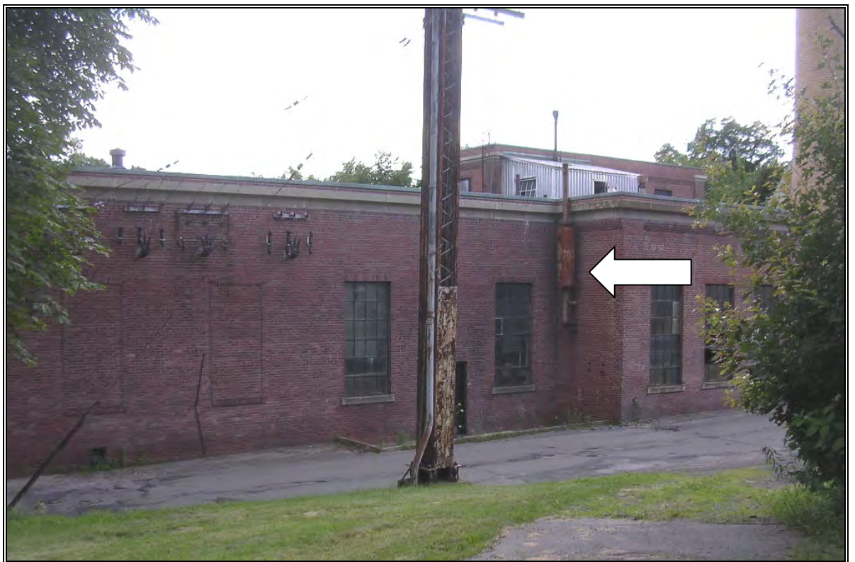
Photo Number 50: Location of generator vent and Power Plant.
