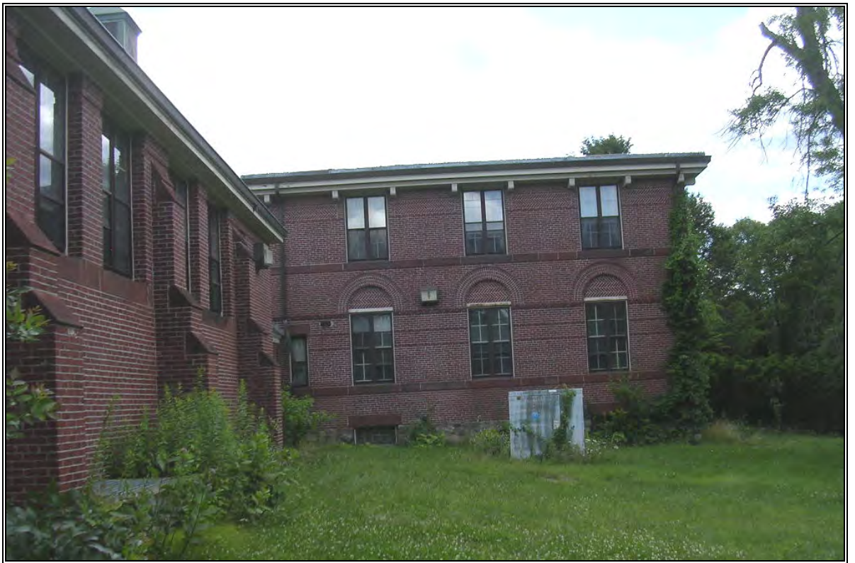
Photo Number 34: Transformer on west side of the Schoolhouse.
