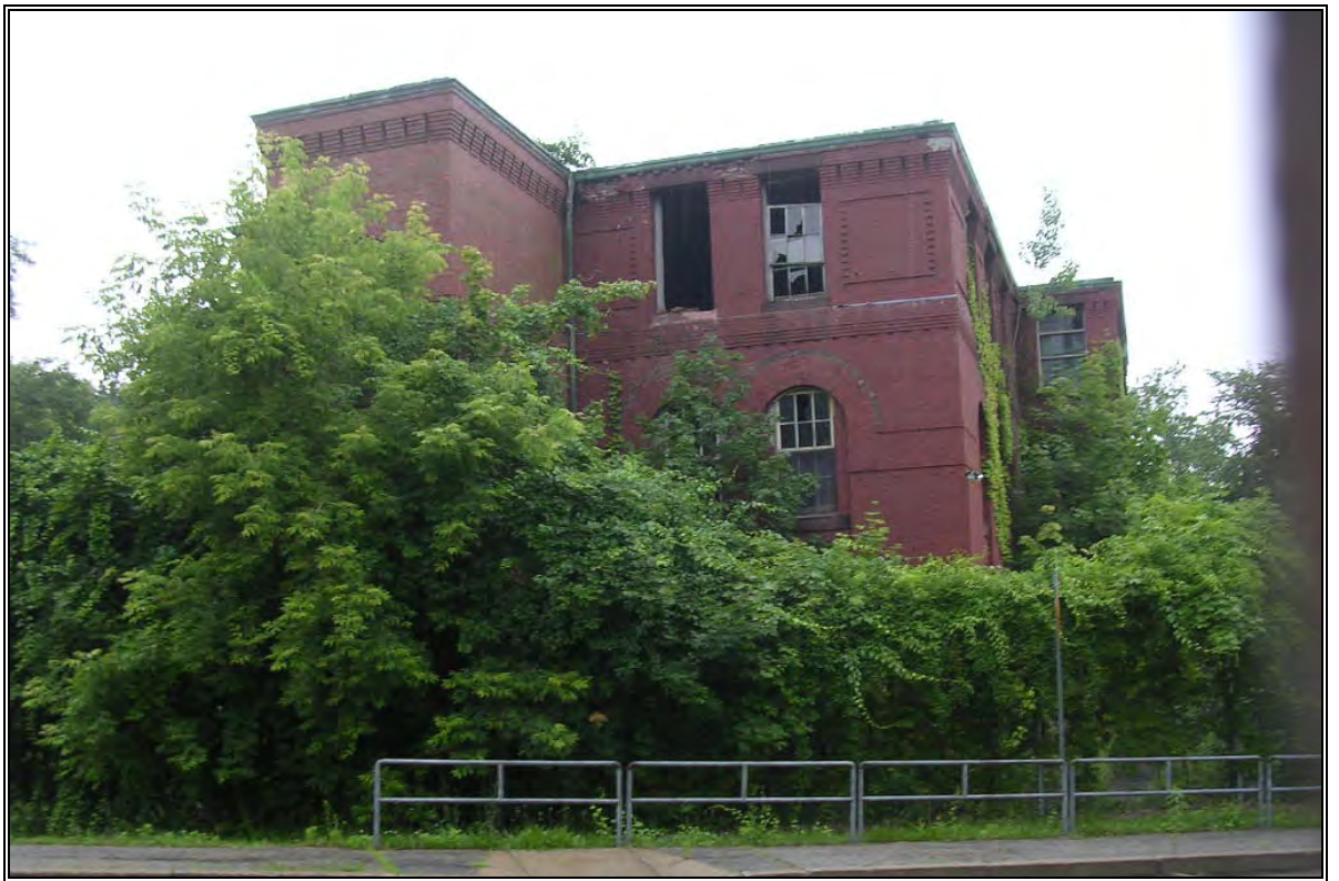
Photo Number 32: East wall of Old Activities Center.
