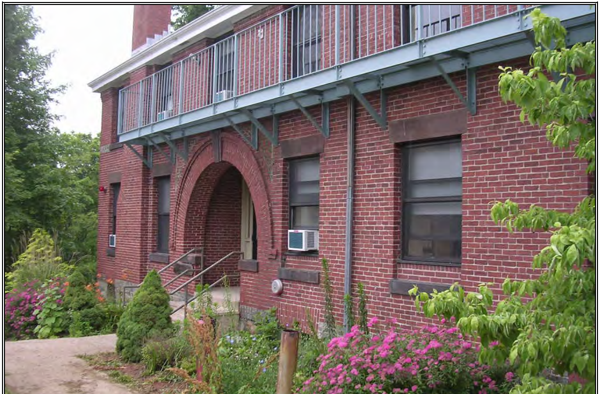
Photo Number 30: South facing wall of North Nurses.
