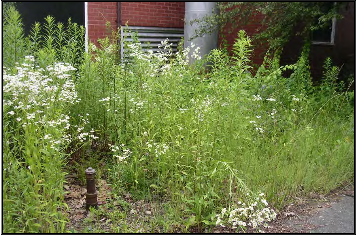
Photo Number 9: UST (7U) fill pipe on north side of Training/New Activities Center.
