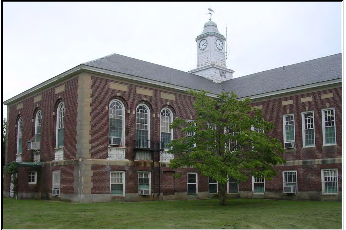
Photo Number 1: North side of Fernald Developmental Center (FDC) Administration Building.
