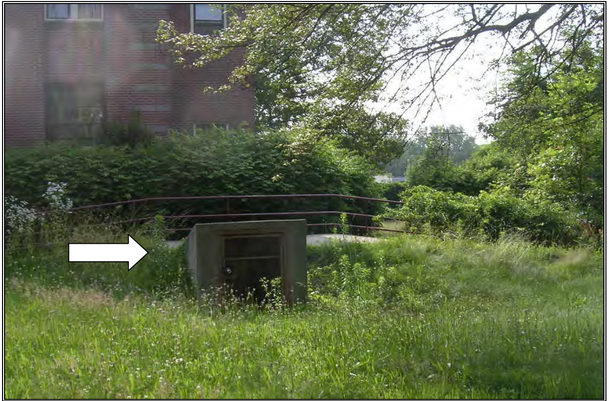
Photo Number 23: Access to steam pipe tunnel near Dolan Hall.
