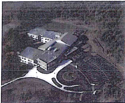
Aerial view, Wood Elementary School, Plainville, Massachusetts
