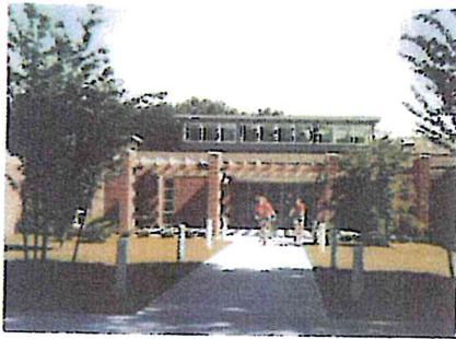
Front Entrance, Hobomock Elementary School, Pembroke, Massachusetts
