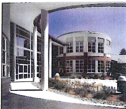
Front Entrance, Salisbury Elementary School, Salisbury, MA
