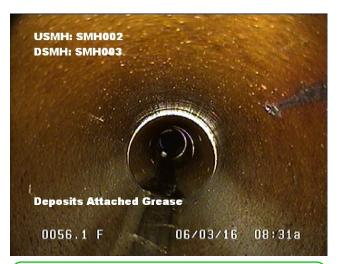
Distance: 55.0 ft. Grade: 2 Condition: **Deposits Attached Grease**
