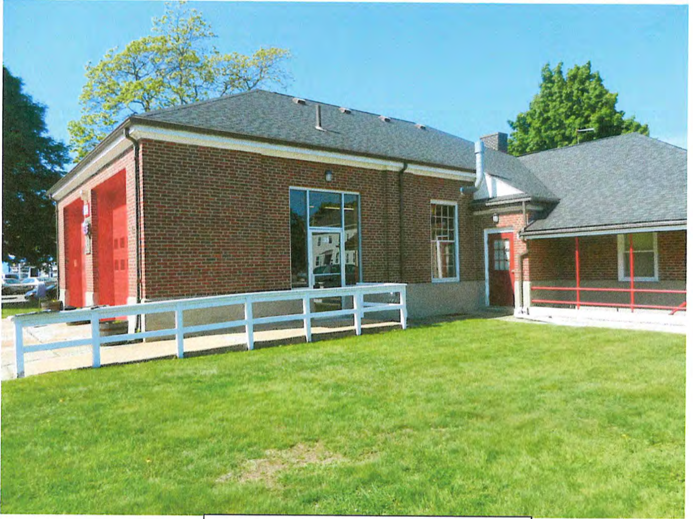
PROSPECT STREET FIRE STATION RIGHT ELEVATION PHOTO-2
