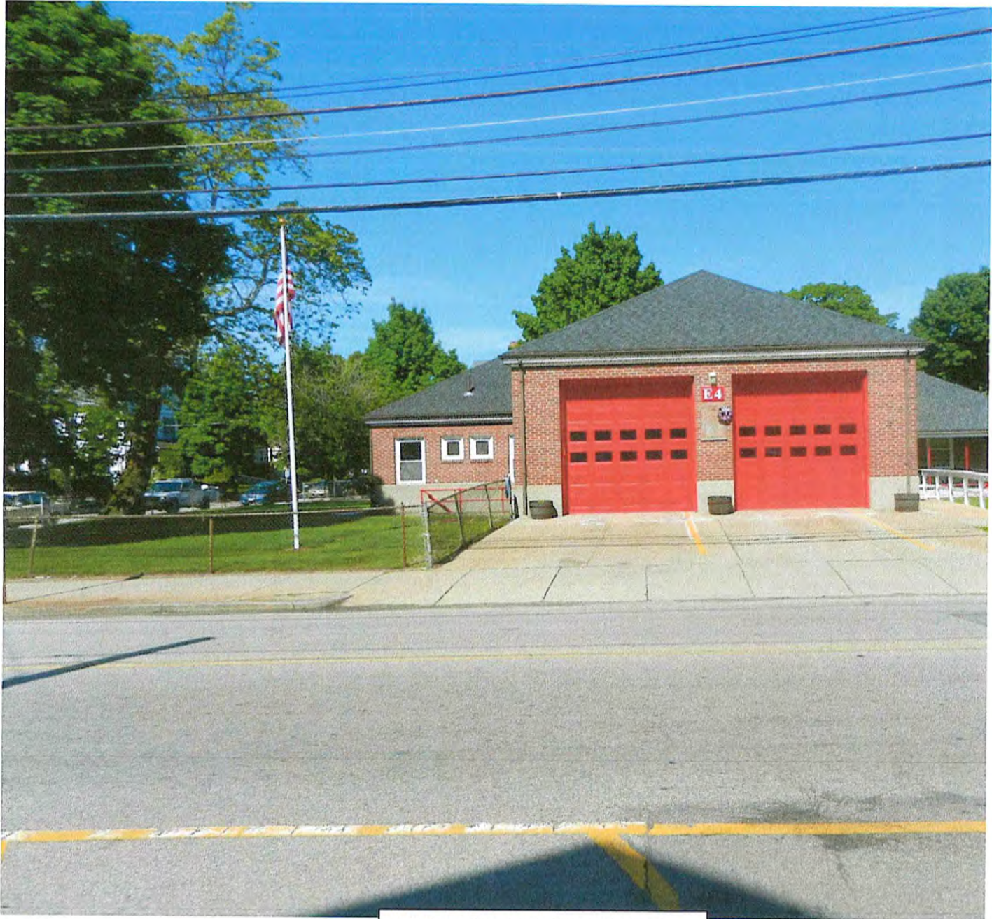
PROSPECT STREET FIRE STATION FRONT ENTRANCE PHOTO- 1
