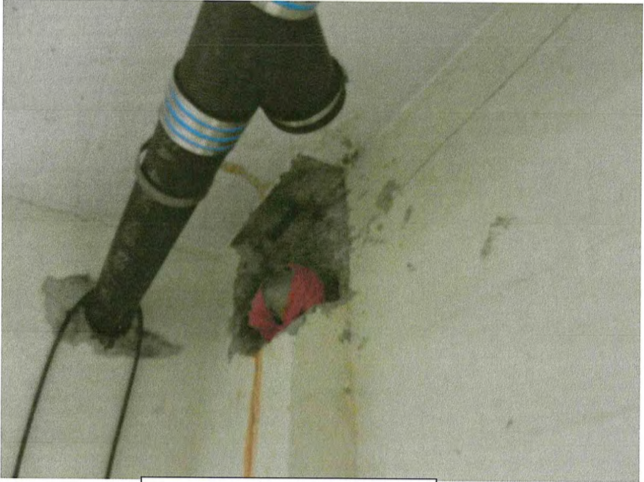
BASEMENT AREA FRONT WALL LEFT SIDE PHOTO-22
