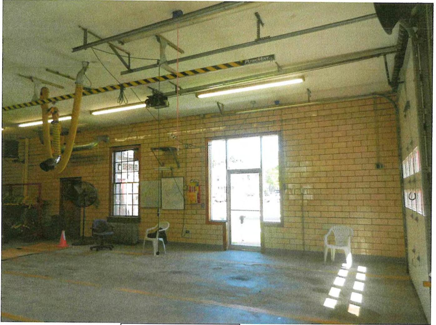
RIGHT SIDE INTERIOR WALL
