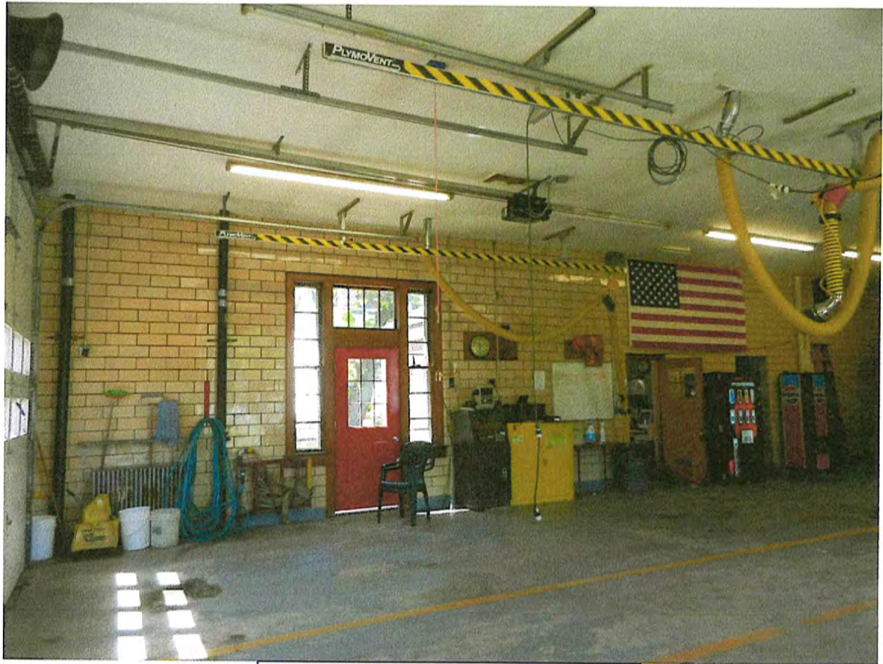
FIRE STATION LEFT SIDE INTERIOR WALL
