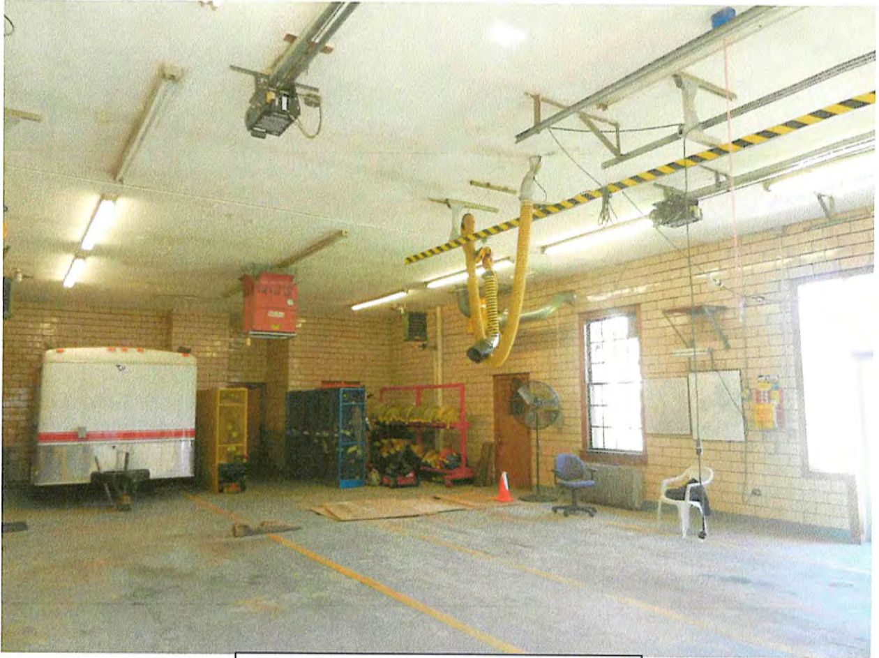
FIRE STATION INTERIOR GARAGE- RIGHT SIDE PHOTO-7
