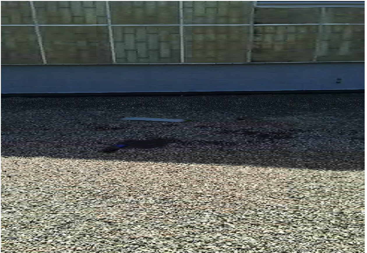
Tar and gravel roof
