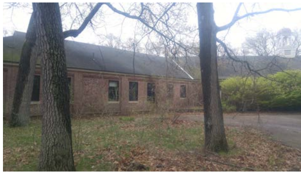
West Building, exterior
