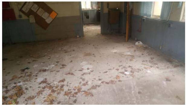
Building 24, floor tile
