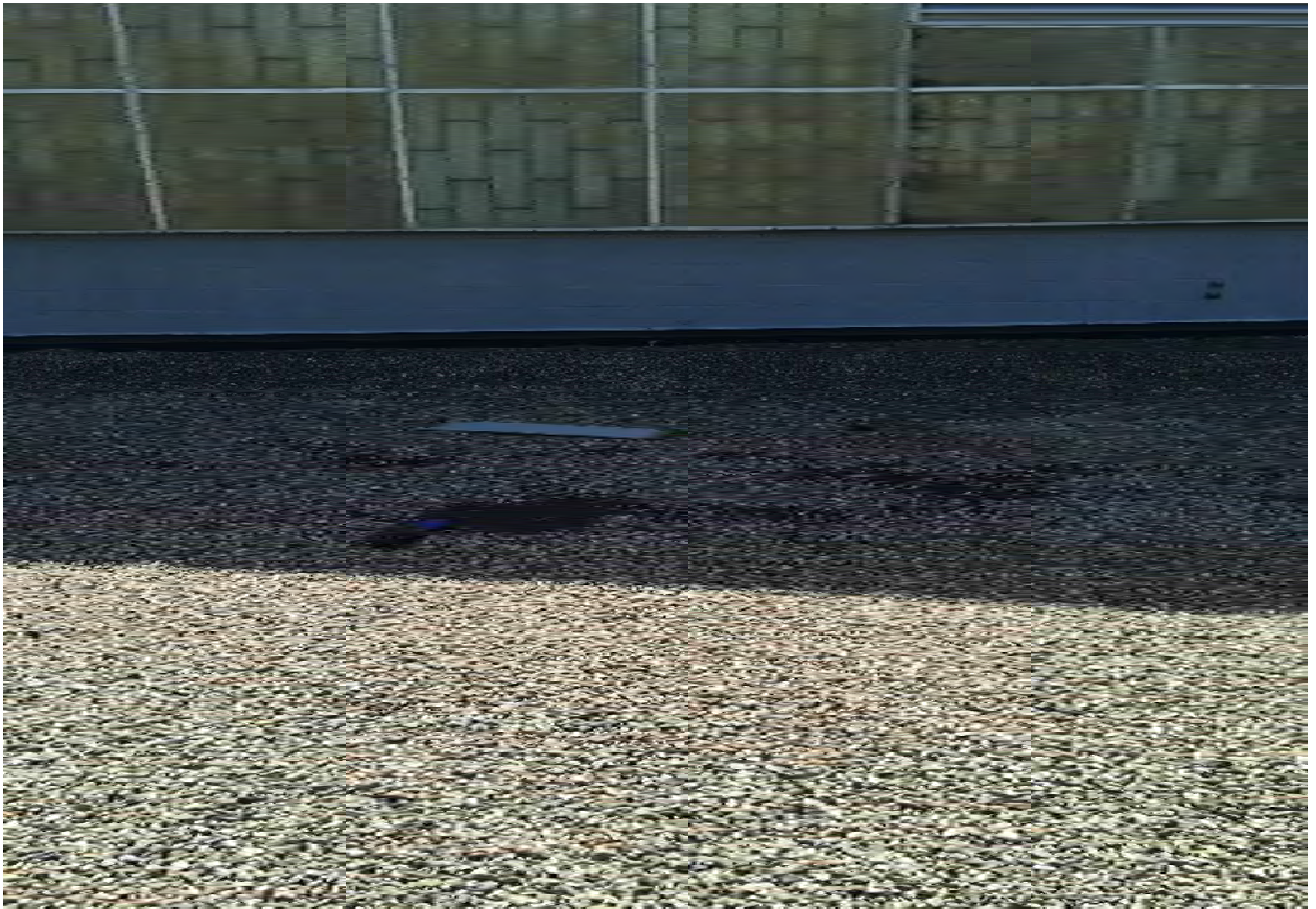
Tar and gravel roof
