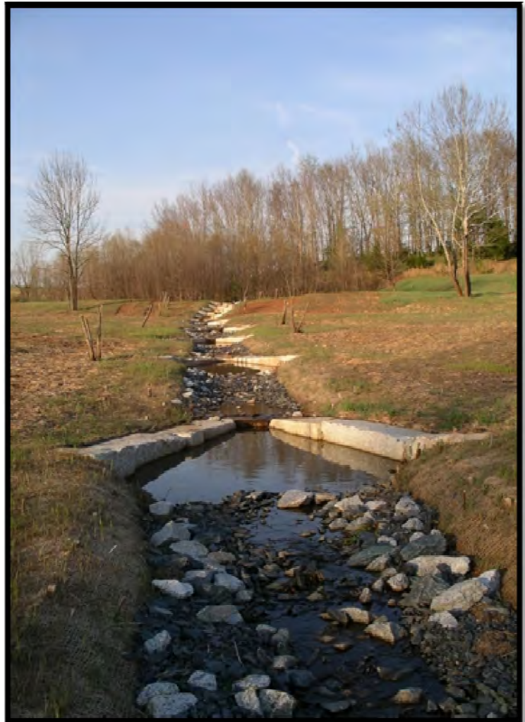
Example of Daylighting a Culvert
