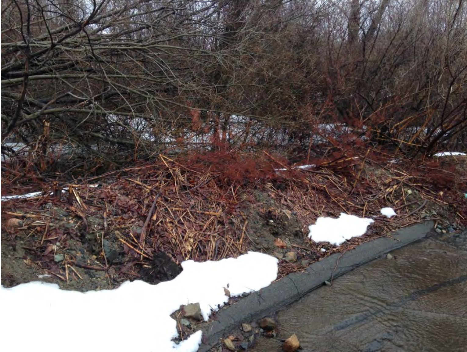
Photo 3 Earthen Berm Installed by the State
