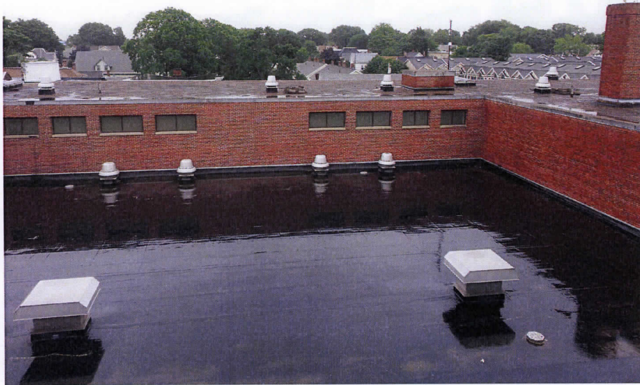
Lower Membrane Roof
