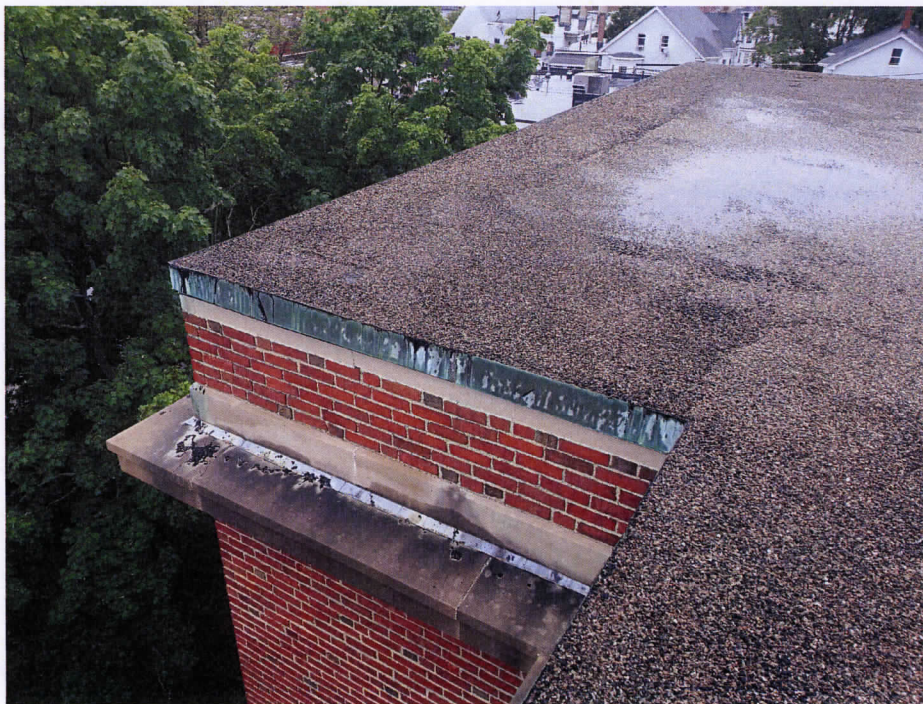
Detail at Built-Up Roof Edge
