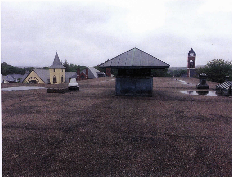
Upper Built-Up Roof over Auditorium
