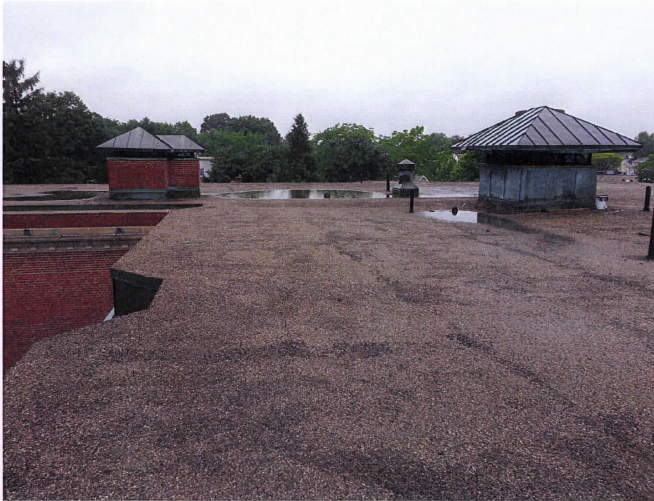
Upper Built-Up Roof Looking South
