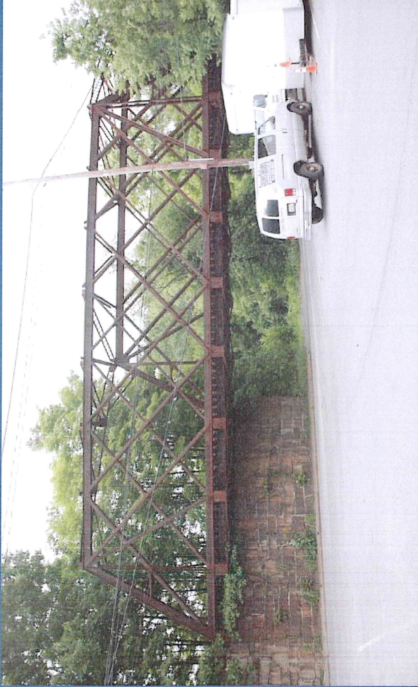
1894, Riveted Lattice Thru Truss Listed on the State Register of Historic Places, Recommended NR eligible
