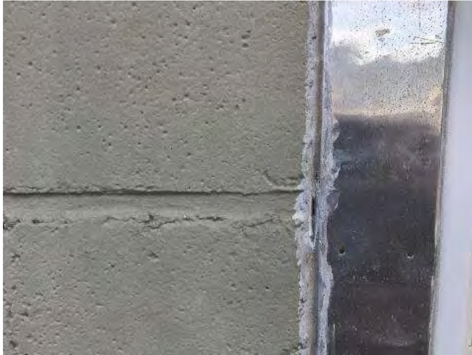
Exterior White Window Caulking
