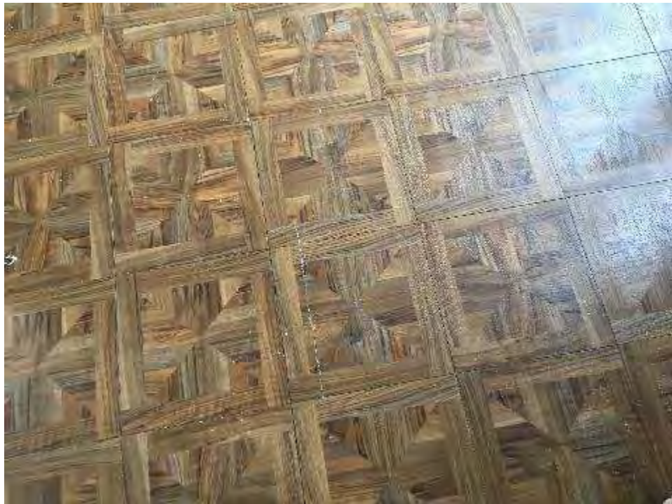
Wood Pattern Stick on Floor Tile and Associated Mastic
