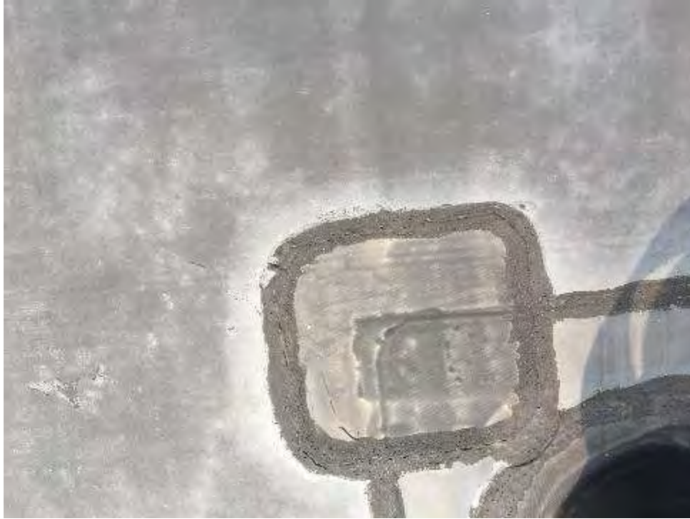
Roof Seam Caulking
