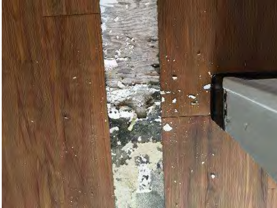
Black Paper Under Tile on Subfloor
