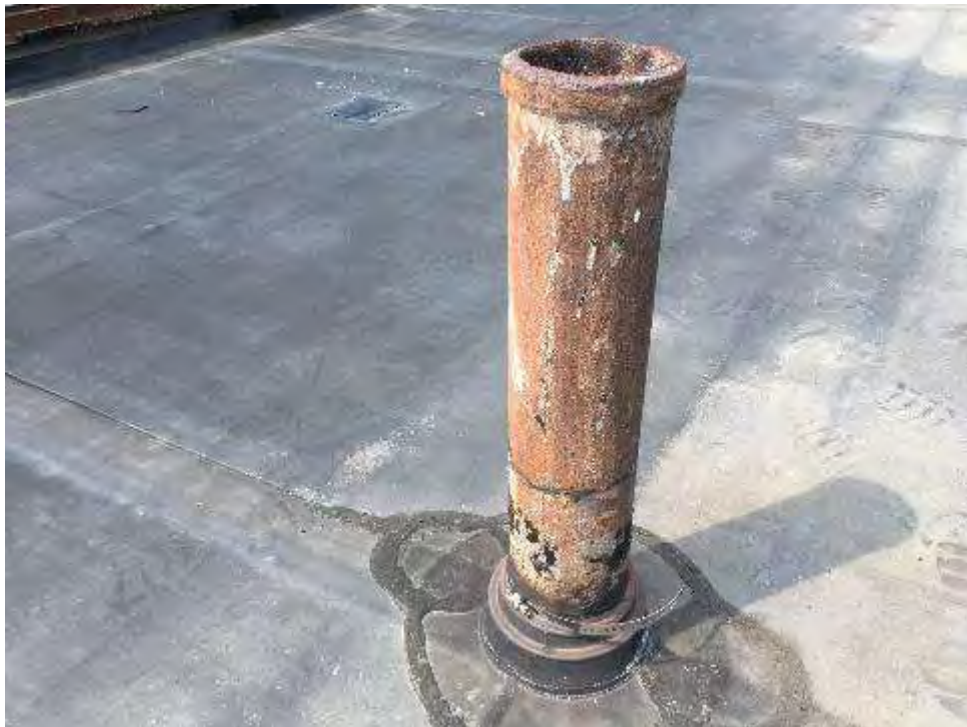
Roof Vent Caulking
