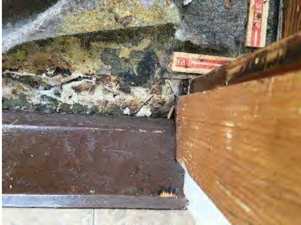
Yellow Capet Pad Mastic, Black Paper and Floor Leveler Compound
