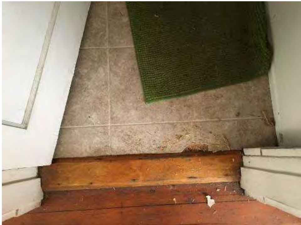
Gray Sheet Flooring and Associated Mastic
