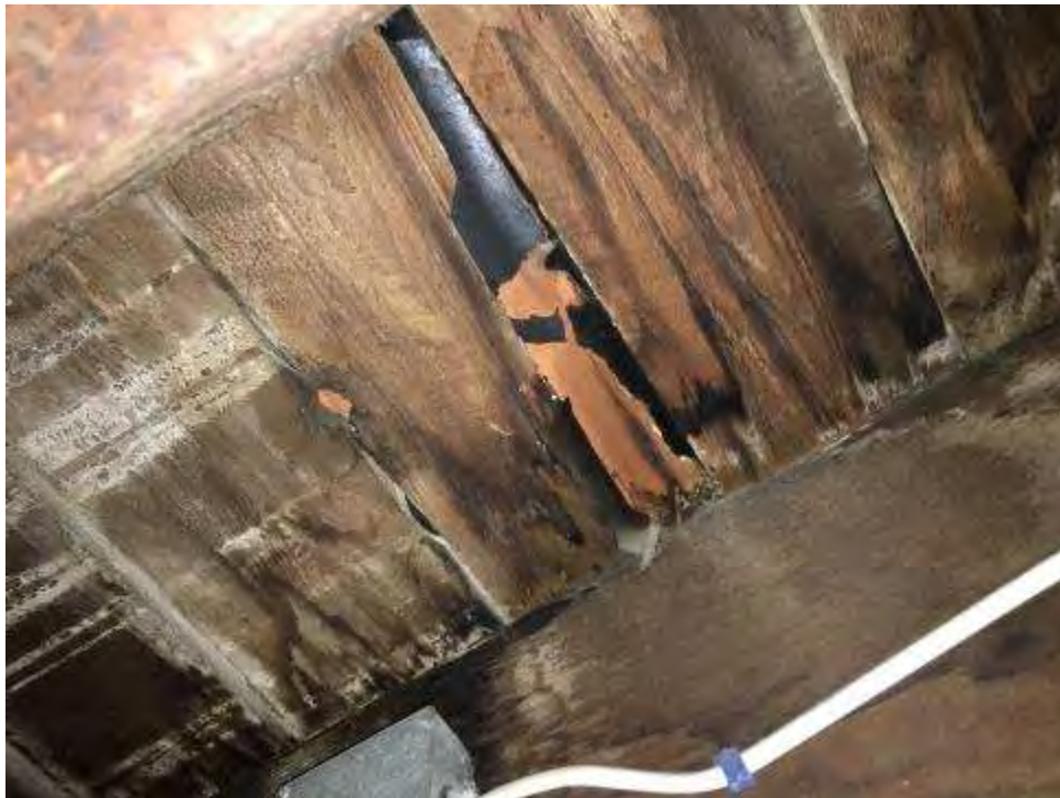
Paper Under 1 st Floor Wood Floor
