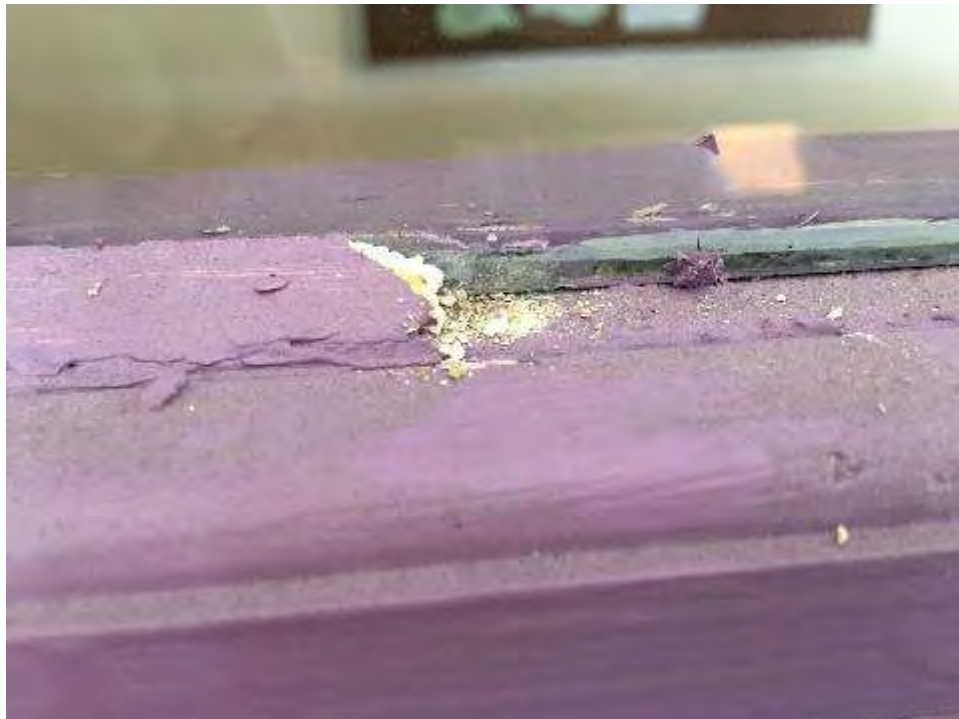
White Interior Window Glazing
