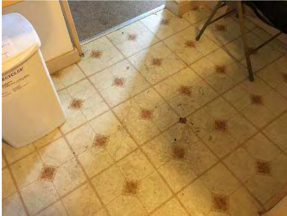
White Square With Brown Diamond Pell and Stick Floor Tile and Associated Mastic
