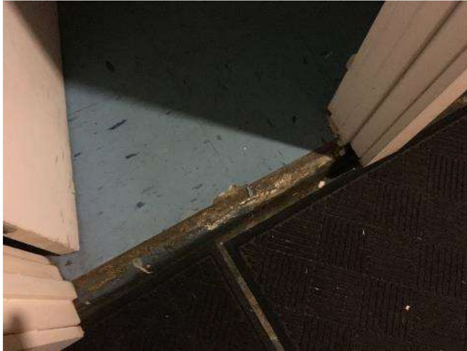
12" x 12" Blue Streak Floor Tile and Associated Mastic
