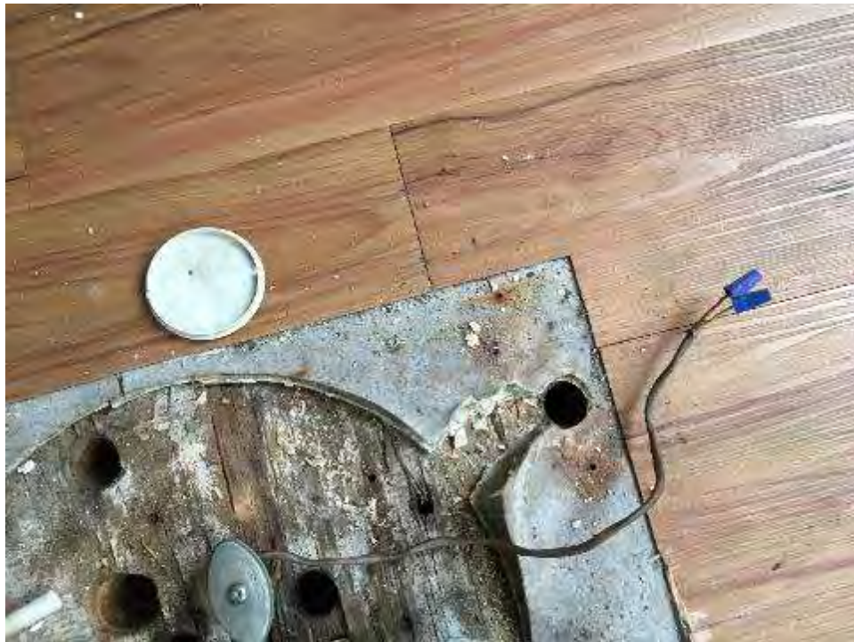
Gray Marble Sheet Flooring Top Layer and Gray Pebble Sheet Flooring Bottom Layer and Associated Mastics
