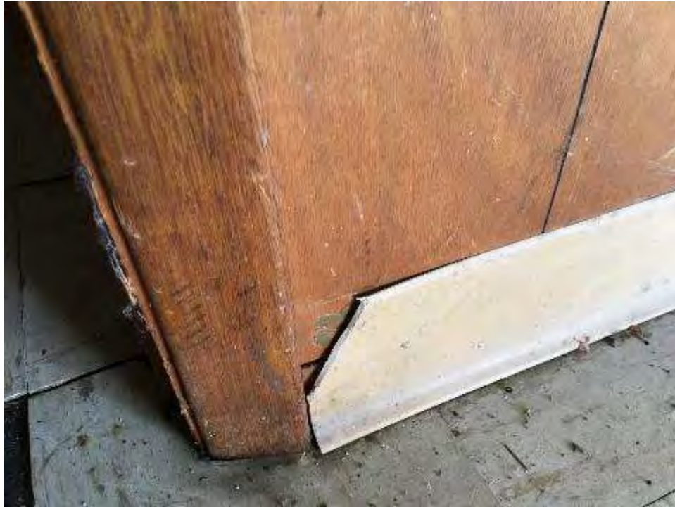
Tan Cove Base and Associated Mastic
