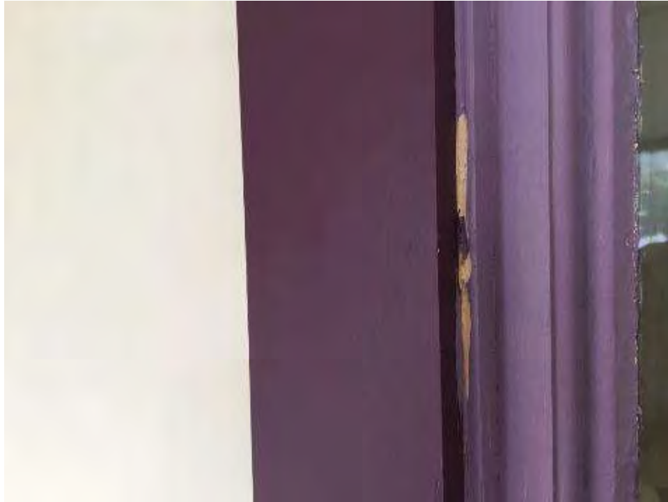
White Interior Window Caulking
