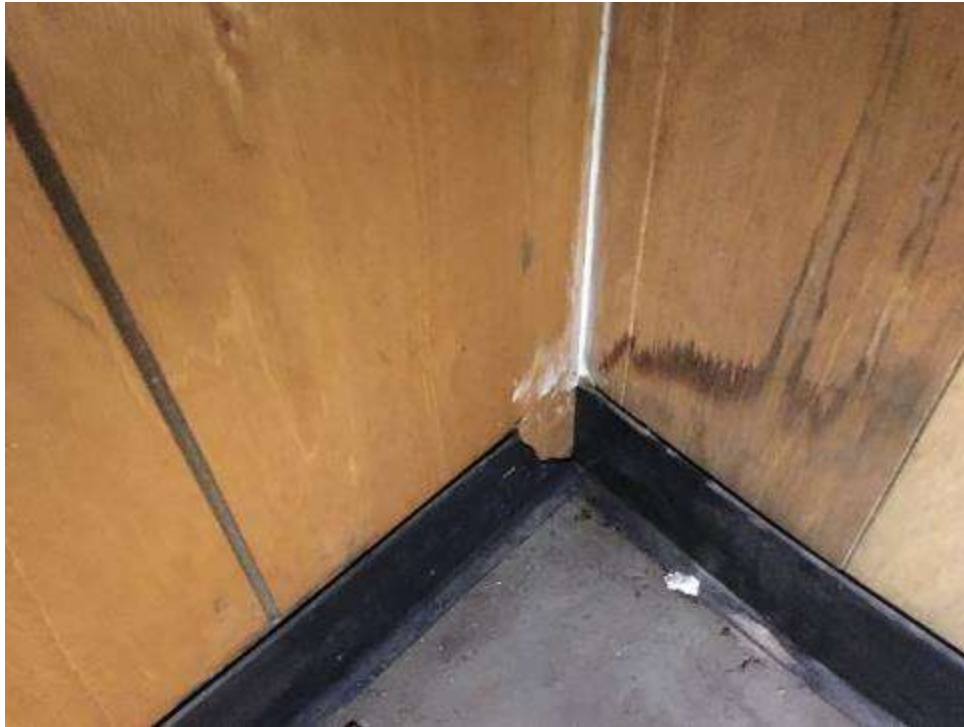
Black Cove Base and Associated Mastic
