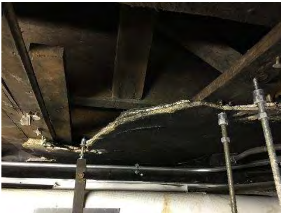
Ceiling Plaster and Backing Sheetrock
