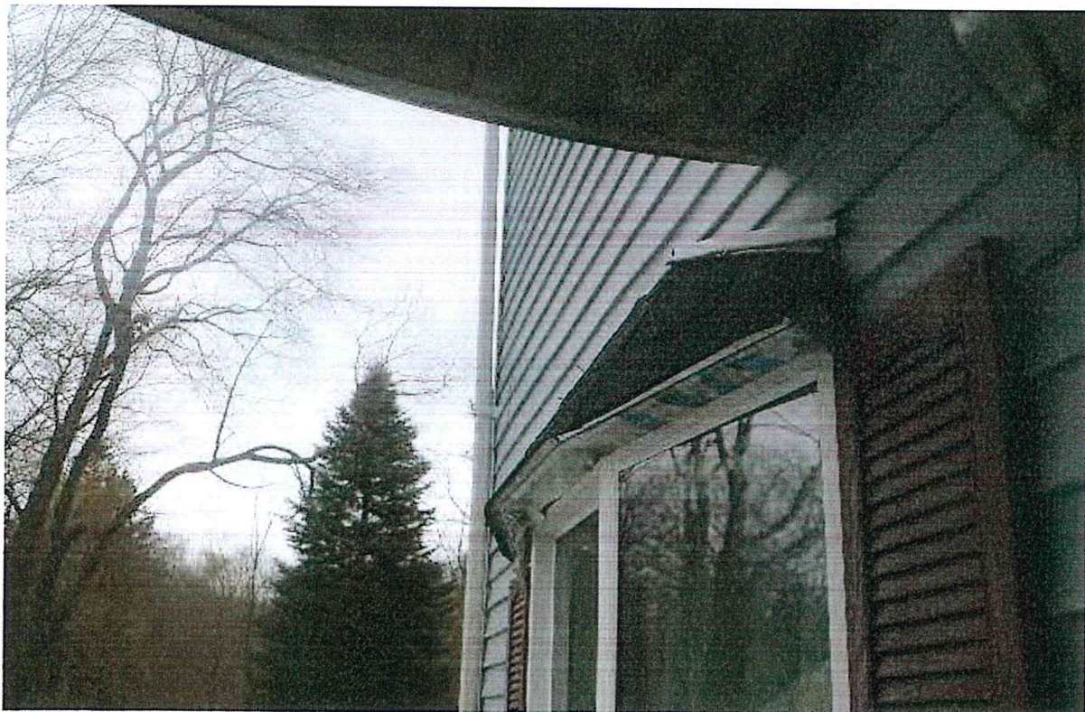
Figure 14: Asphalt roof shingles
