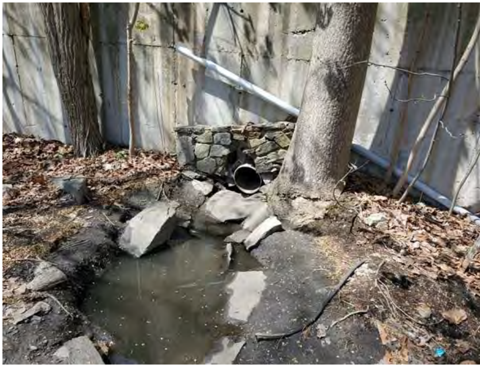
Photo 5: Culvert near flag A-132.
