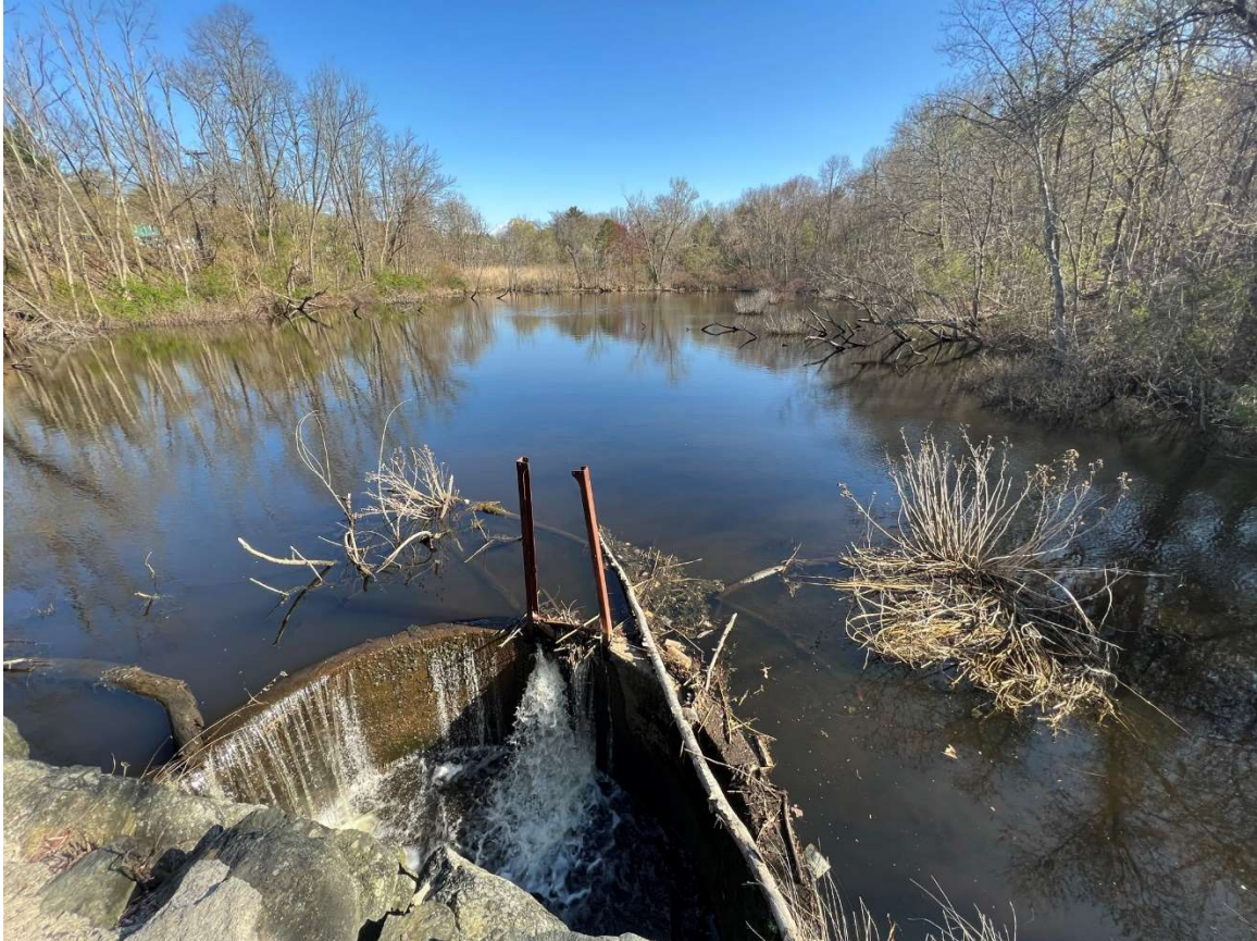
Figure 24. Chester Brook YMCA Wetland Existing Outlet Structure
