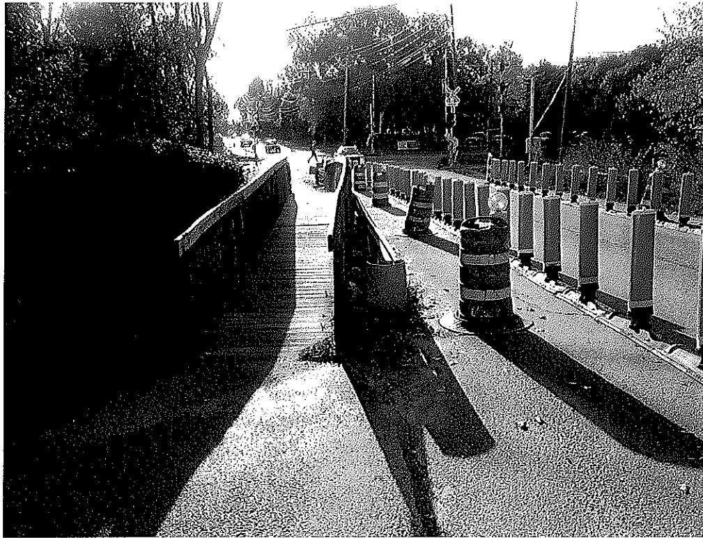
Photo 5: Traffic has been restricted from driving over the steel plates located on the East side of the culvert
