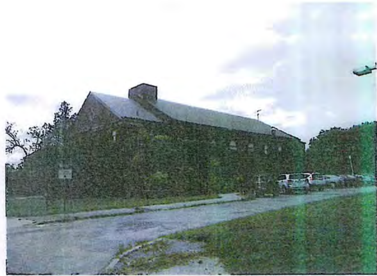
136. View West of East and North Elevations of Howe Hall
