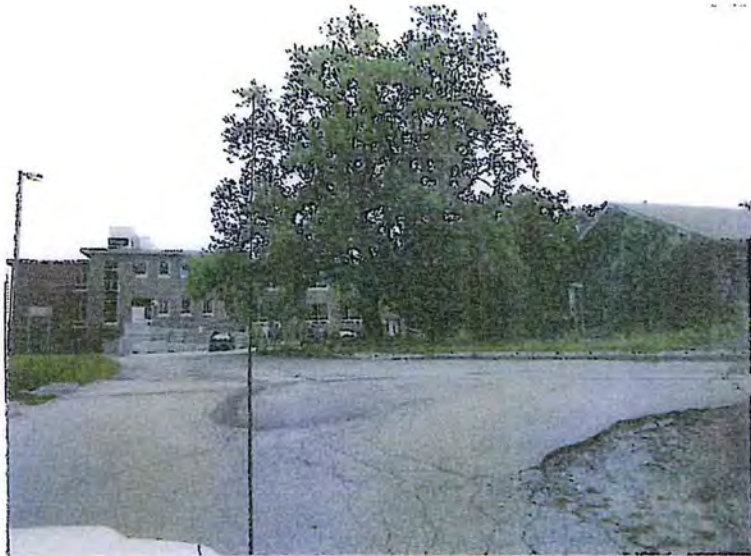
147. View West of East Elevation of Greene Unit
