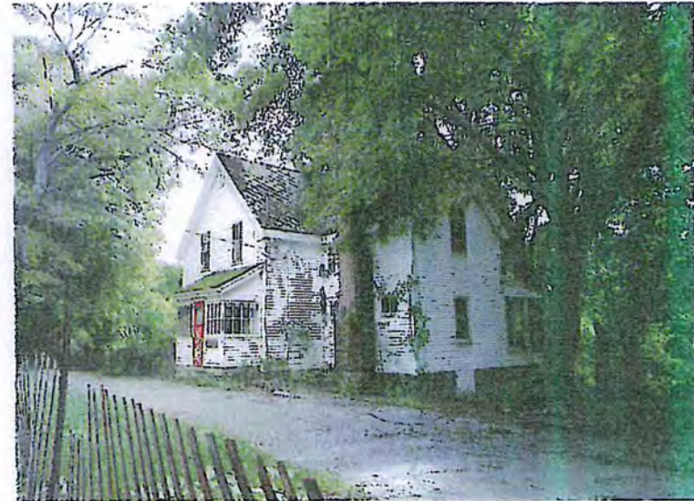
138. View Southwest of East and North Elevations of Baldwin Cottage
