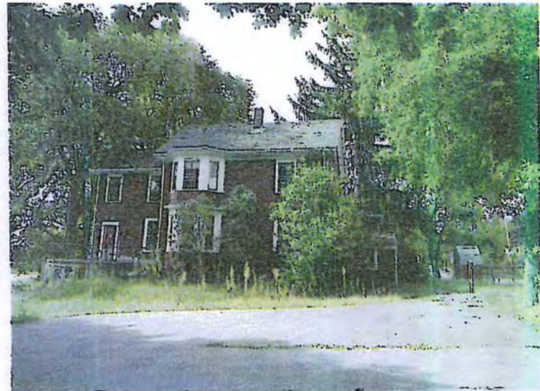
150. View West of East Elevation of Trapelo Cottage
