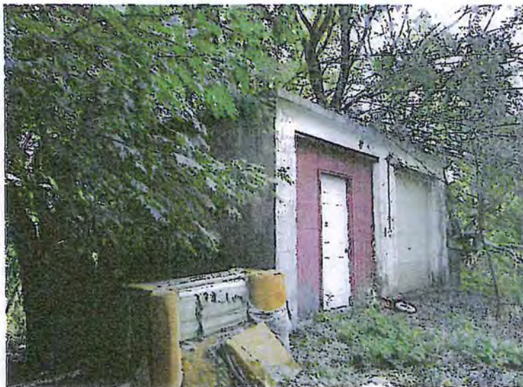
153. View North of South and East Elevations of Cardinal Cottage Garage
