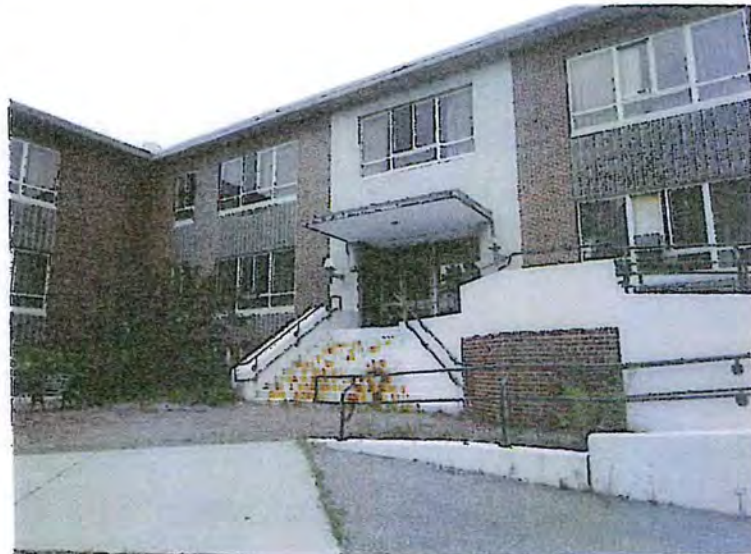
149. View North of South Elevation of Greene Unit
