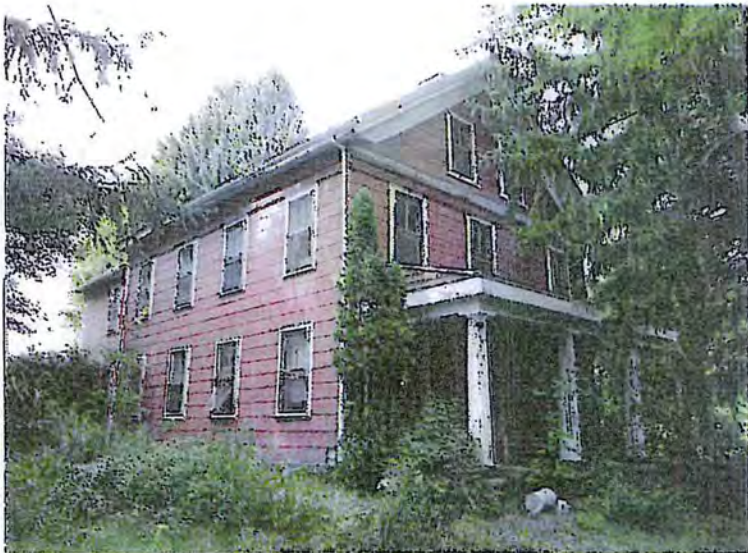
151. View North of South and East Elevations of Cardinal Cottage
