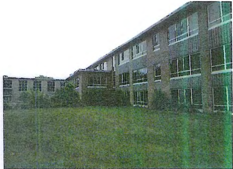
148. View Southeast of West and North Elevations of Greene Unit
