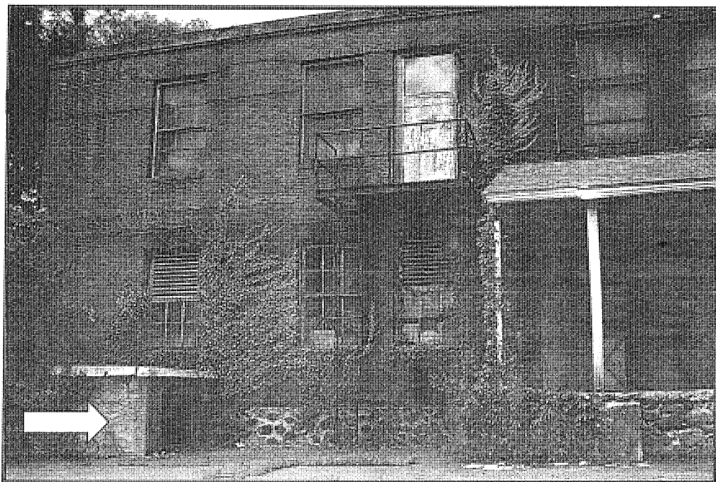
Photo Number 40: Southwest wall of Store Room and open steam pipe vault (on left).
