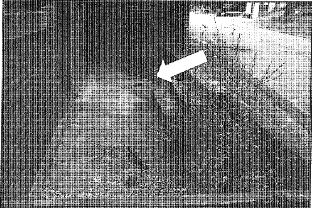
Photo Number 51: Former location of gasoline UST (formerly used for Power Plant generator)
