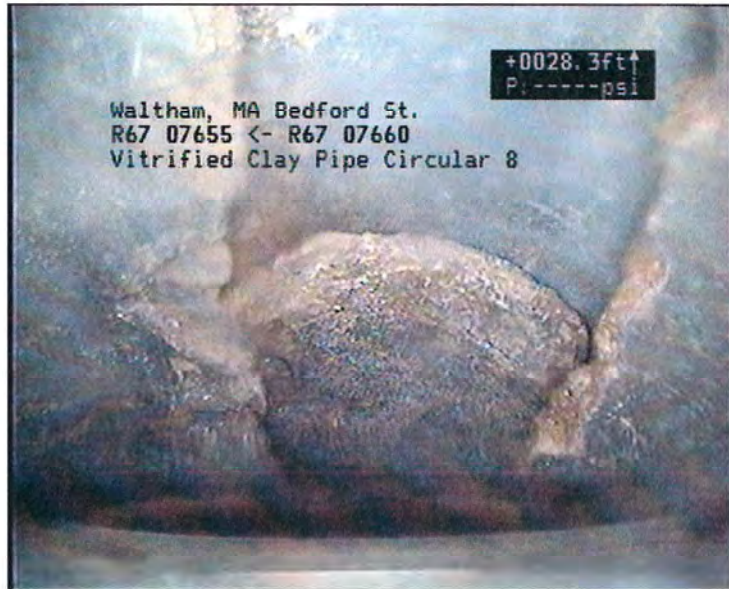
Photo: 59_60_296_A.JPG, VCR No.: Waltham TV #2 28.1FT, Hole, from 10 to 02 o'clock, within 8 inches of joint: YES
