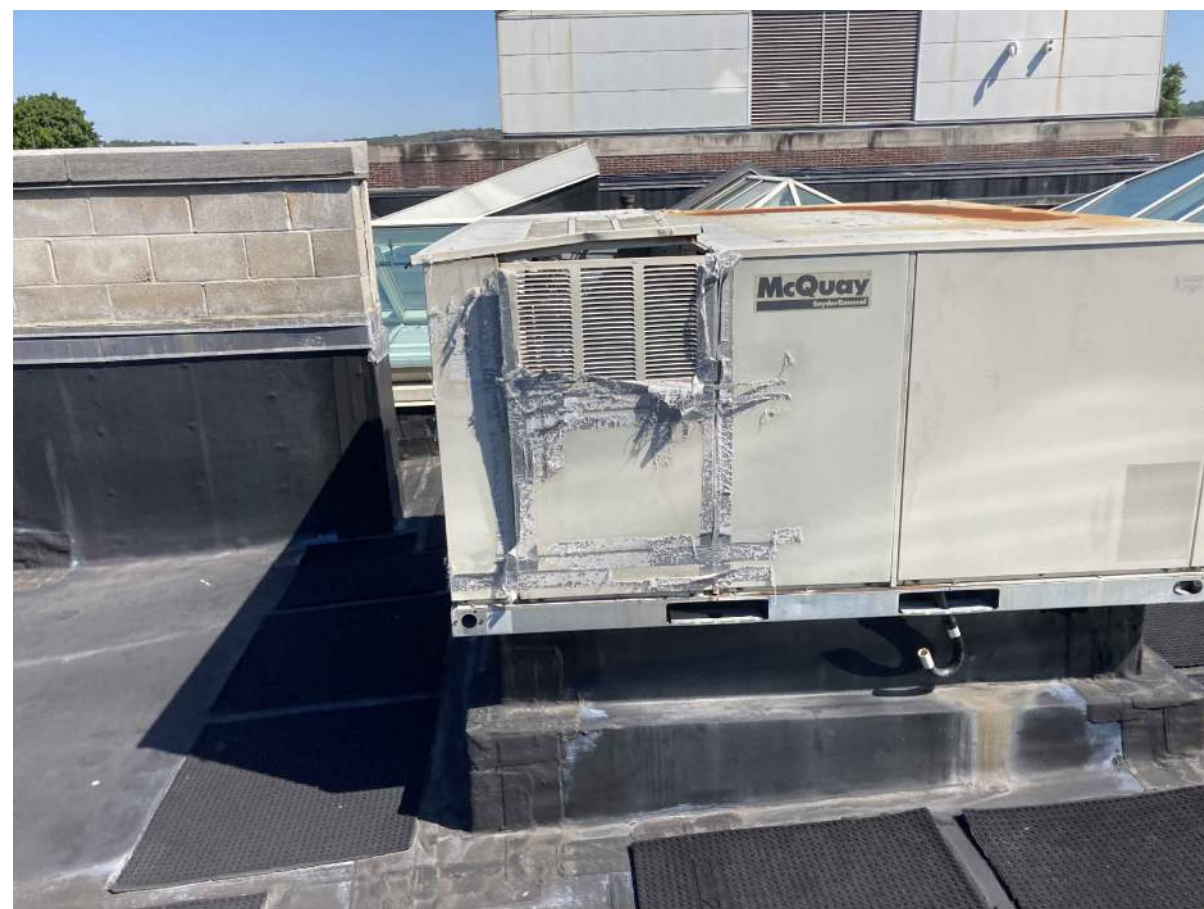
PHOTOGRAPH NO. 5 EXISTING ROOFTOP UNIT (RTU-5) TO BE REMOVED.
