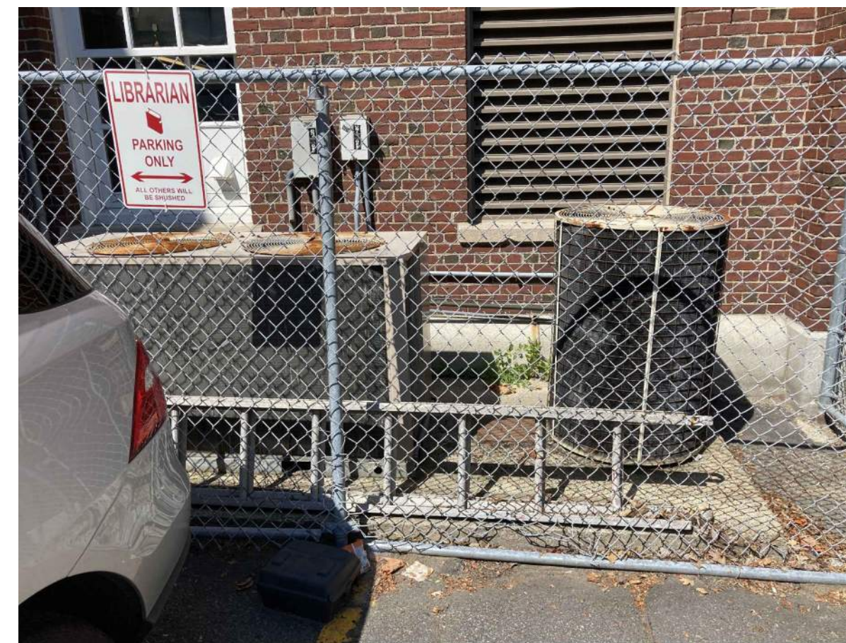
PHOTOGRAPH NO. 7 EXISTING GRADE MOUNTED CONDENSING UNITS TO BE REMOVED.
