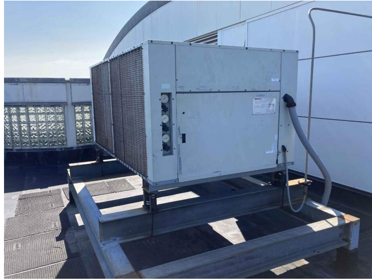
PHOTOGRAPH NO. 1 EXISTING CONDENSING UNIT TO BE REMOVED.
