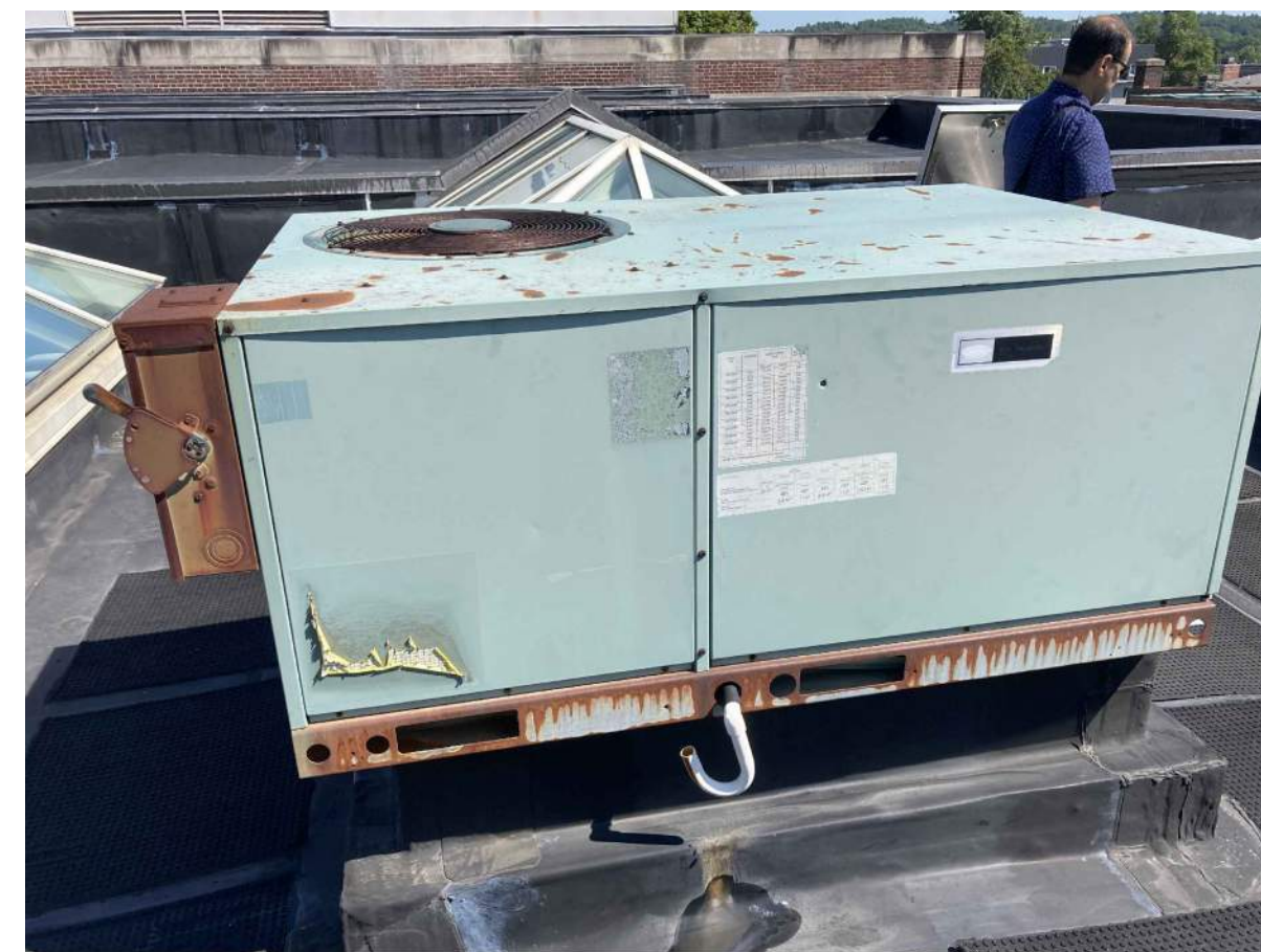
PHOTOGRAPH NO. 6 EXISTING ROOFTOP UNIT (RTU-6) TO BE REMOVED.
