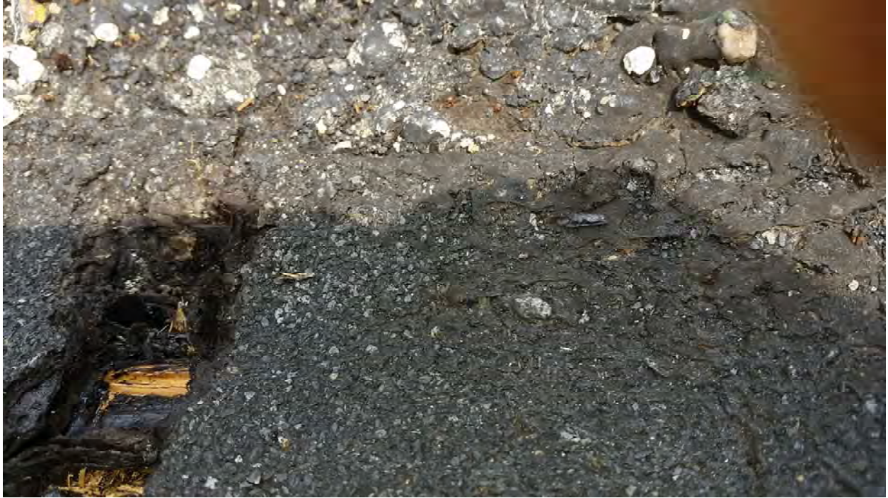
Black main field roof tar
