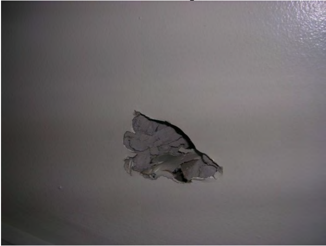
HA's 44,45,46 Sheetrock, Joint Compound, Joint Tape – 2 nd
