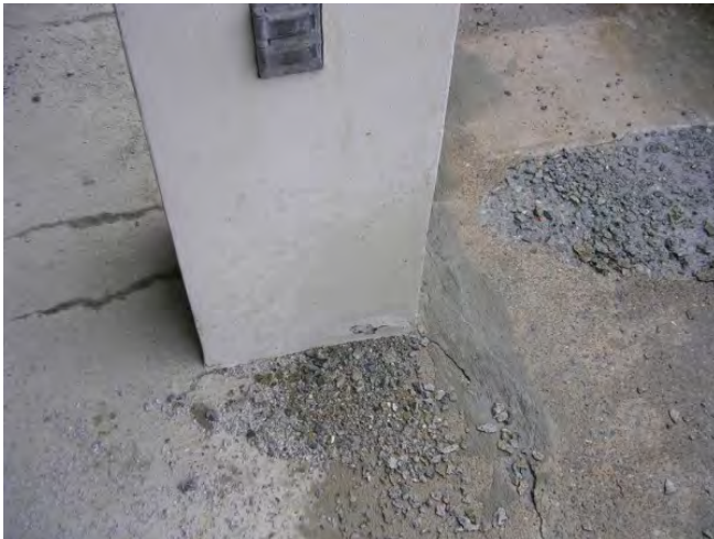
HA 84 Skim Coat (textured) on Concrete Columns, Exterior
