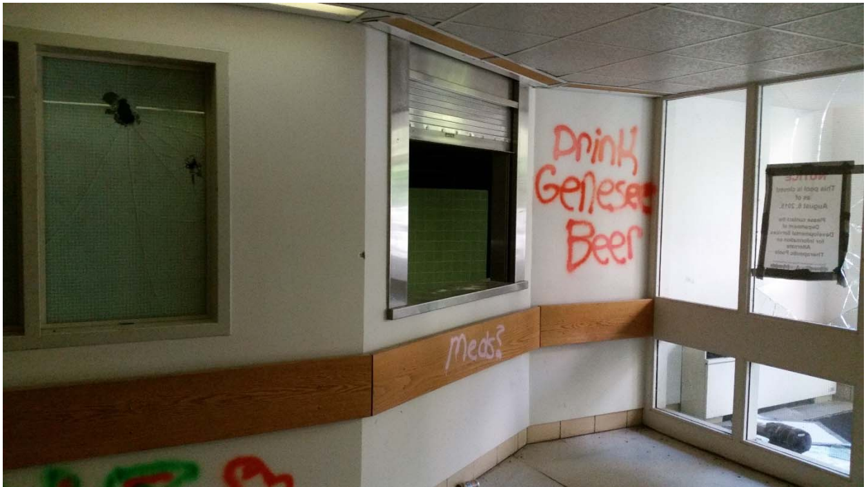
Sheetrock and joint compound walls
