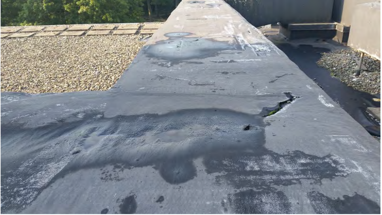
Black duct covering
