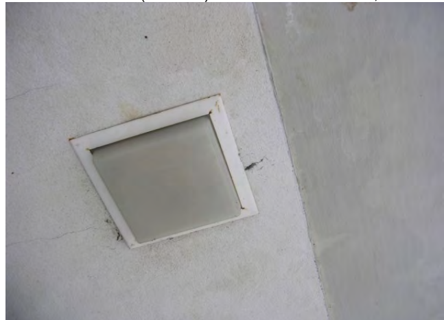
HA 86,87 Plaster at Front Entry, Skim and Base Coats
