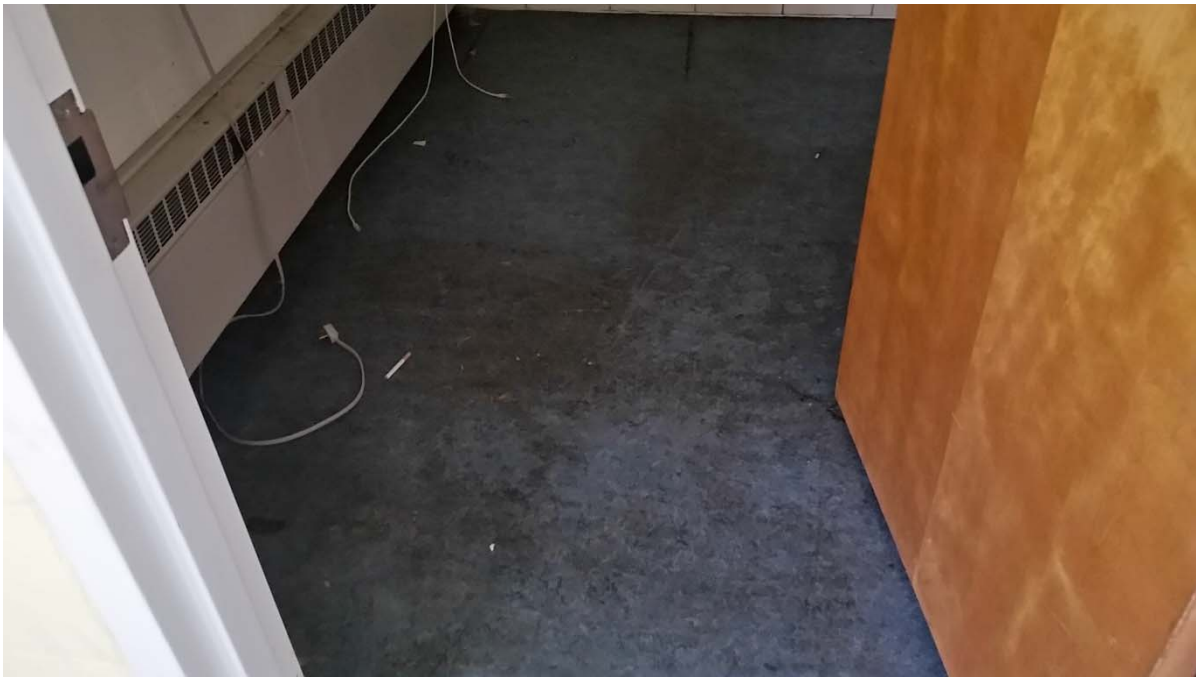
Blue sheet flooring and associated white mastic
