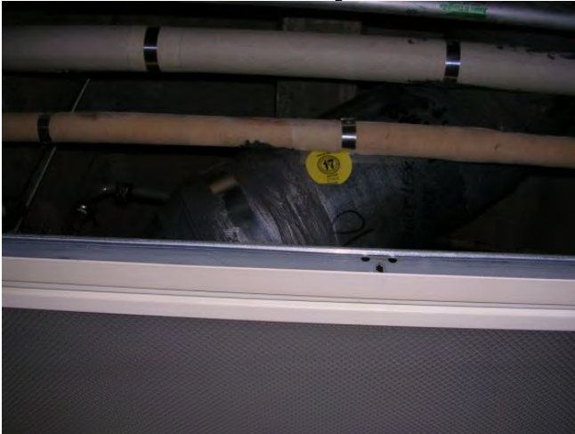
HA 54 Grey HVAC Seam Sealant
