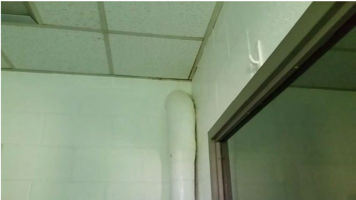
ACM pipe fitting insulation
