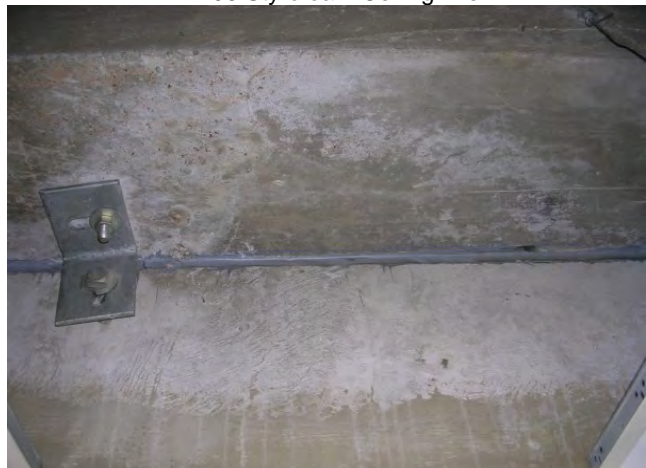
HA 98 Gray Caulk at Roof Deck
