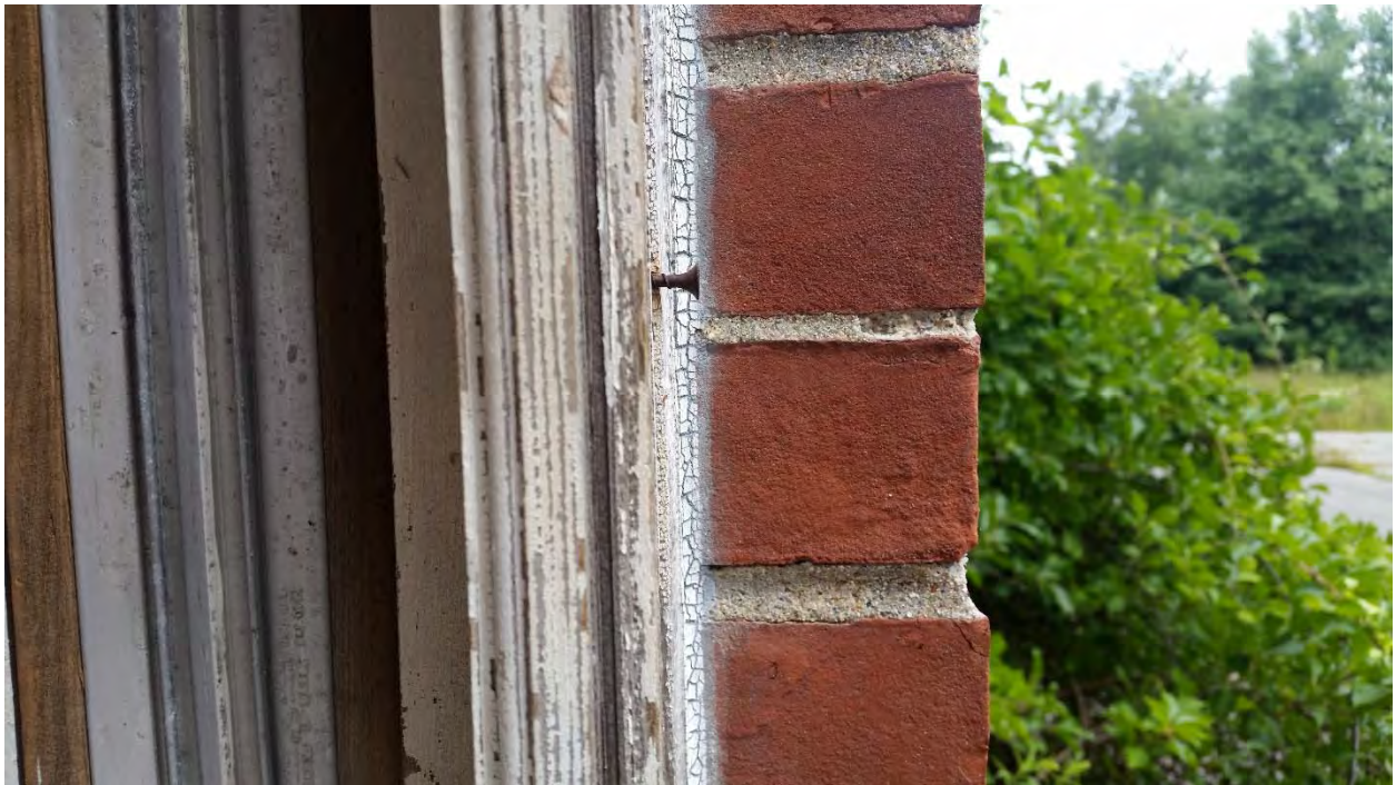
Grey exterior window caulk
