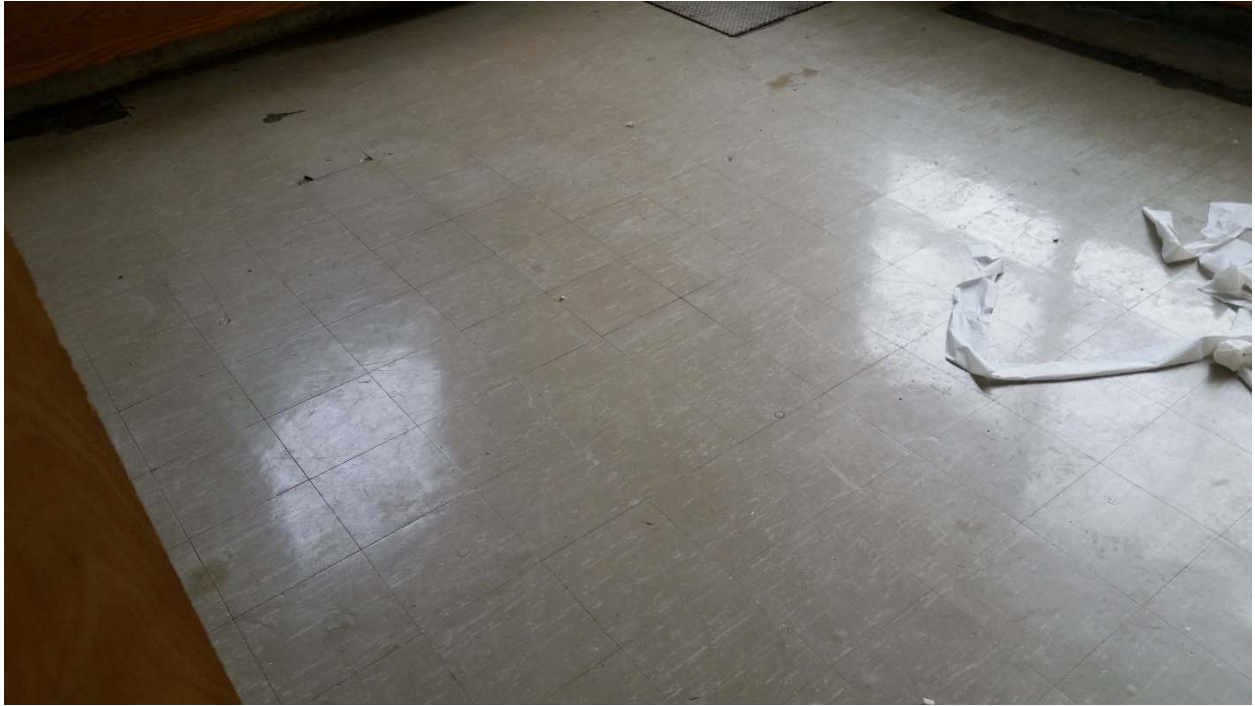
ACM 9"x9" grey floor tile and associated ACM black mastic
