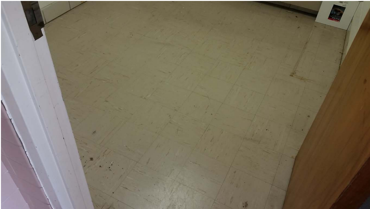
ACM 9"x9" tan floor tile and associated ACM black mastic
