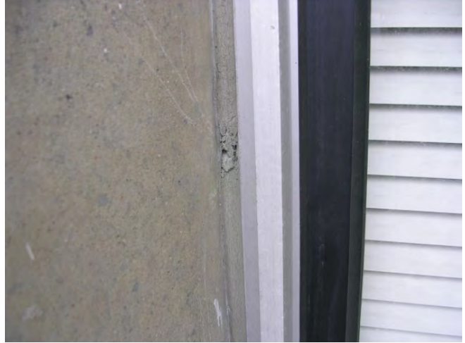
HA 82,83 Window Caulking (Grey), Window Glazing (black)
