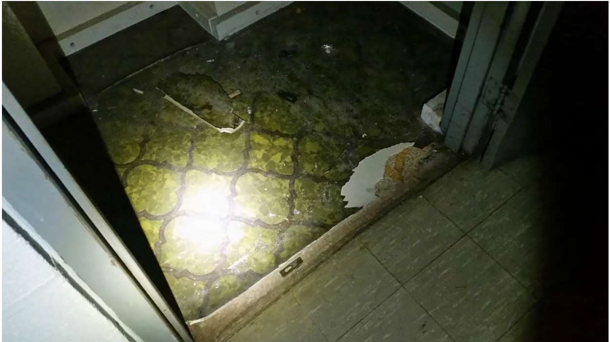
ACM green linoleum and associated non-ACM backing
