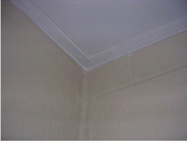
HA 101 White Caulk on Ceiling Grid
