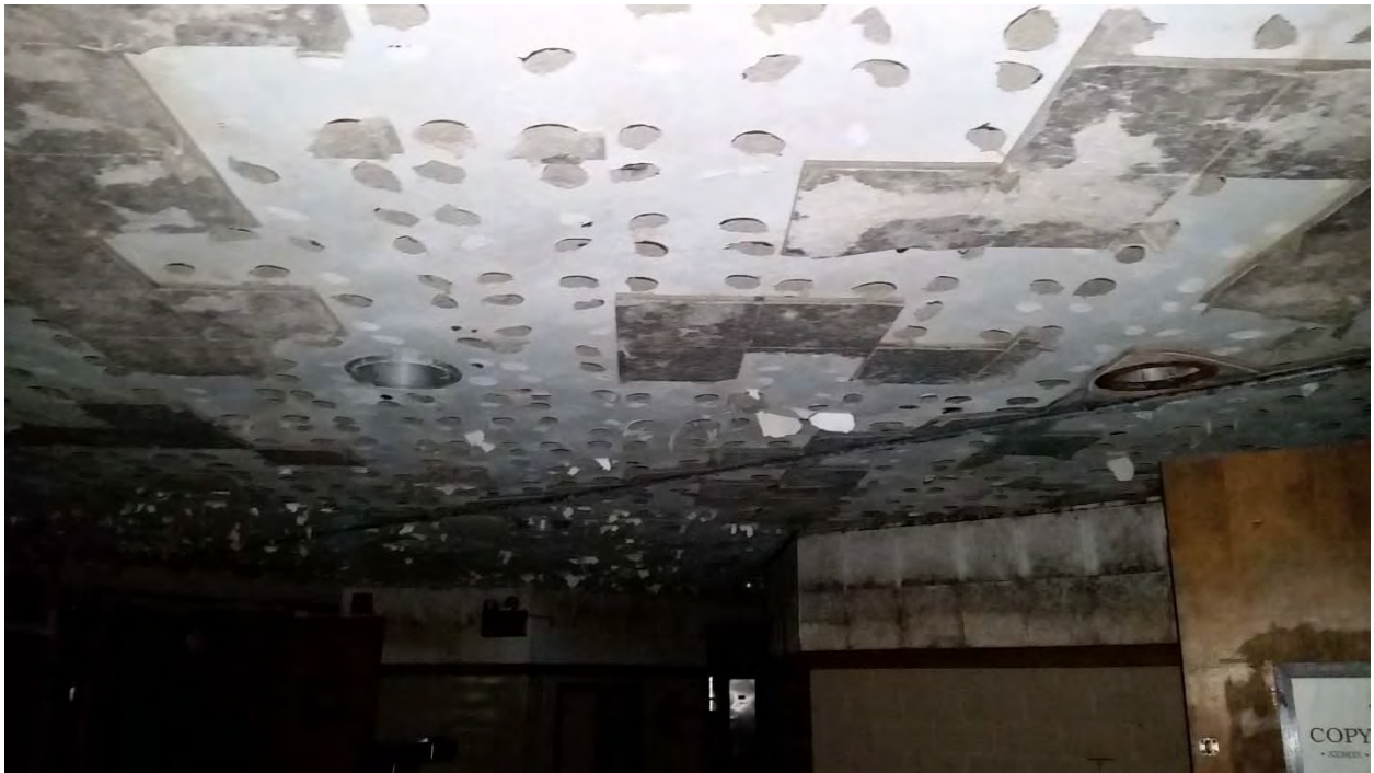
1'x1' white squiggle ceiling tiles and associated glue daubs.
