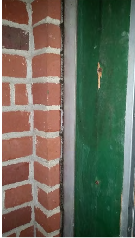
ACM exterior door caulk, and non-ACM brick and mortar
