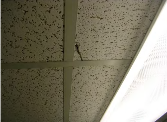
HA's 04,05 2'x4' Ceiling Tile, White Speck and Fissured
