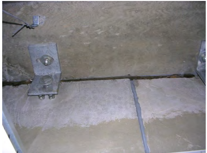
HA 97 Brown Caulk at Roof Deck
