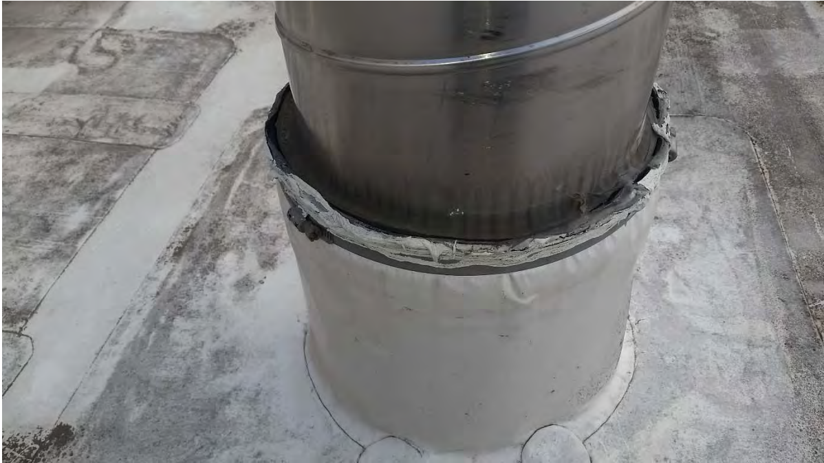
White penetration sealant
