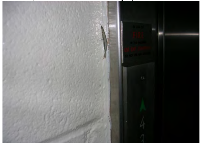
HA 53 Caulking around Elevator
