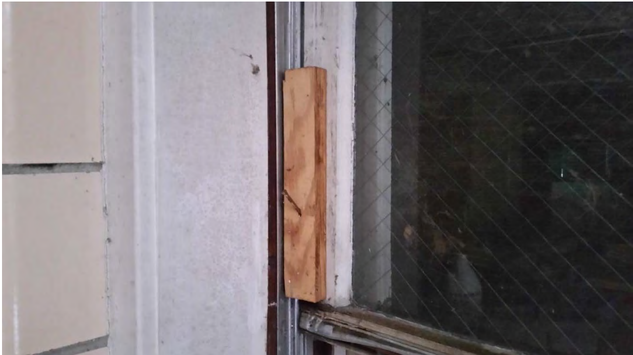
ACM Interior window glazing (Note- most windows were removed and stored in the Window Storage Room on the 1 st Floor)
