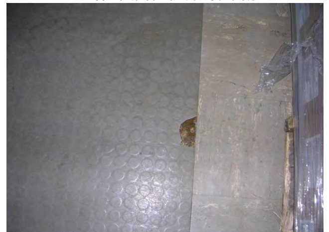
HA's 72,73 Rubber Flooring and Mastic
