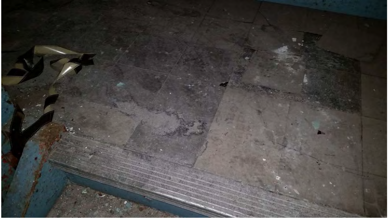
ACM 9"x9" grey floor tile and associated non-ACM black mastic
