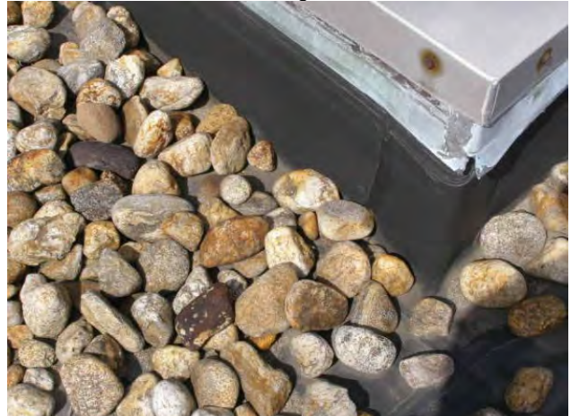
HA 09 Black Caulk on Roof Vents
