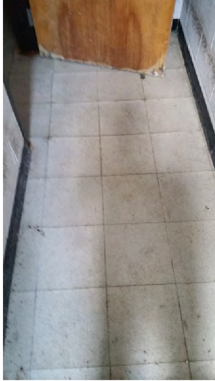
12"x12" grey dot floor tile and associated mastic
