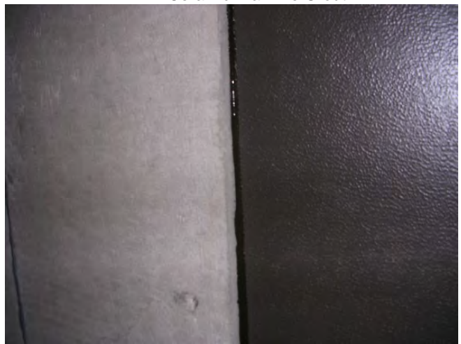
HA 29 Glue/Caulk around Metal Window Panels
