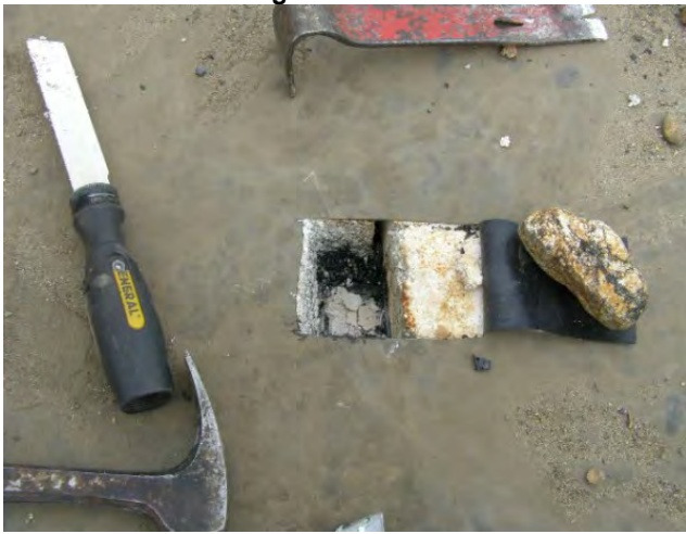
HA's 89, 91 Tar & Gravel Roofing Tars/Felts, Gypsum Roof
