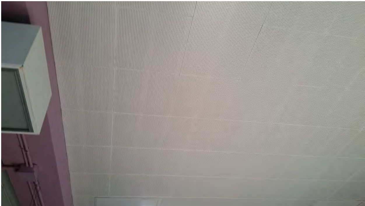
ACM 2'x2' pinhole cementitious ceiling tiles
