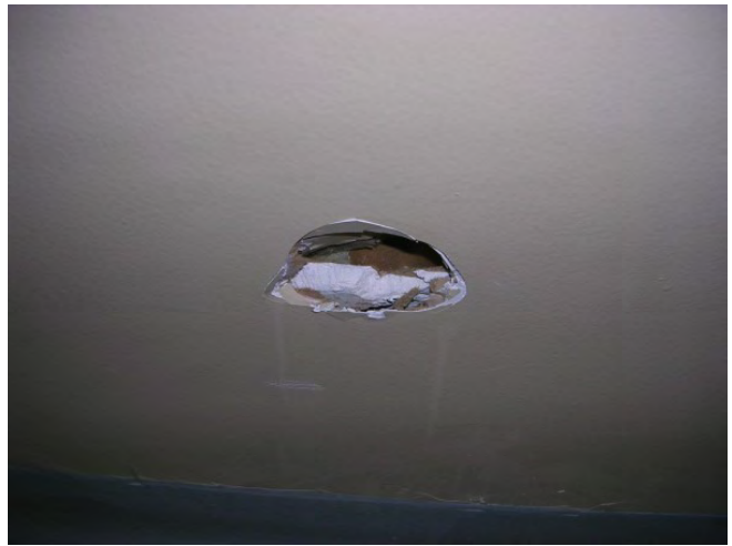
HA's 02, 03, 04 Sheetrock, Joint Compound, Joint Tape – 4th Floor
