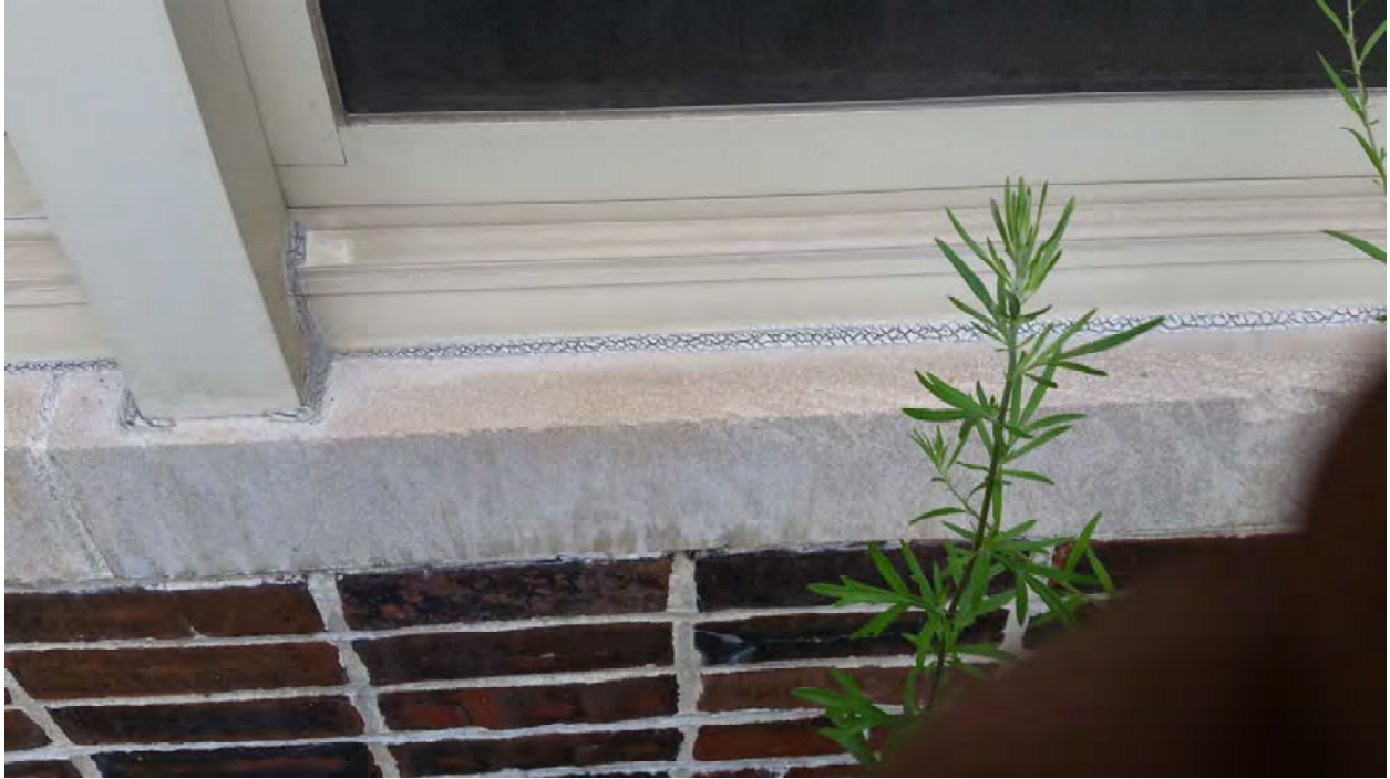
Exterior white window caulk, brick, and mortar
