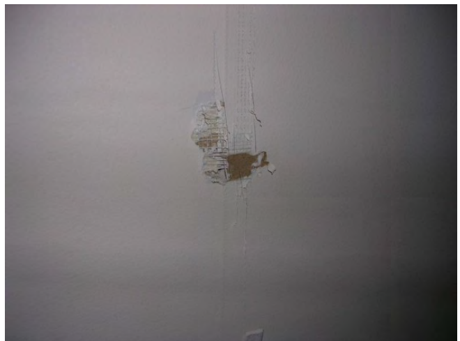
HA's 23,24,25 Sheetrock, Joint Compound, Joint Tape – 3 rd
