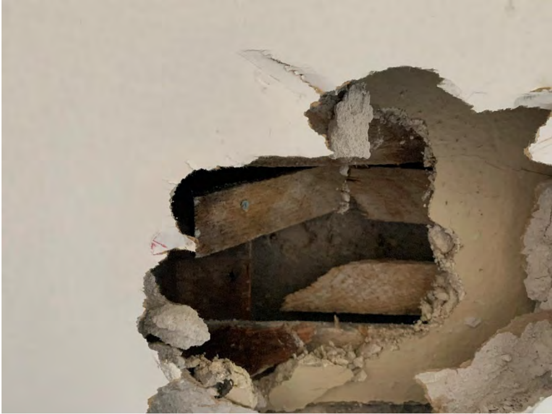
Plaster wall behind gypsum wall
