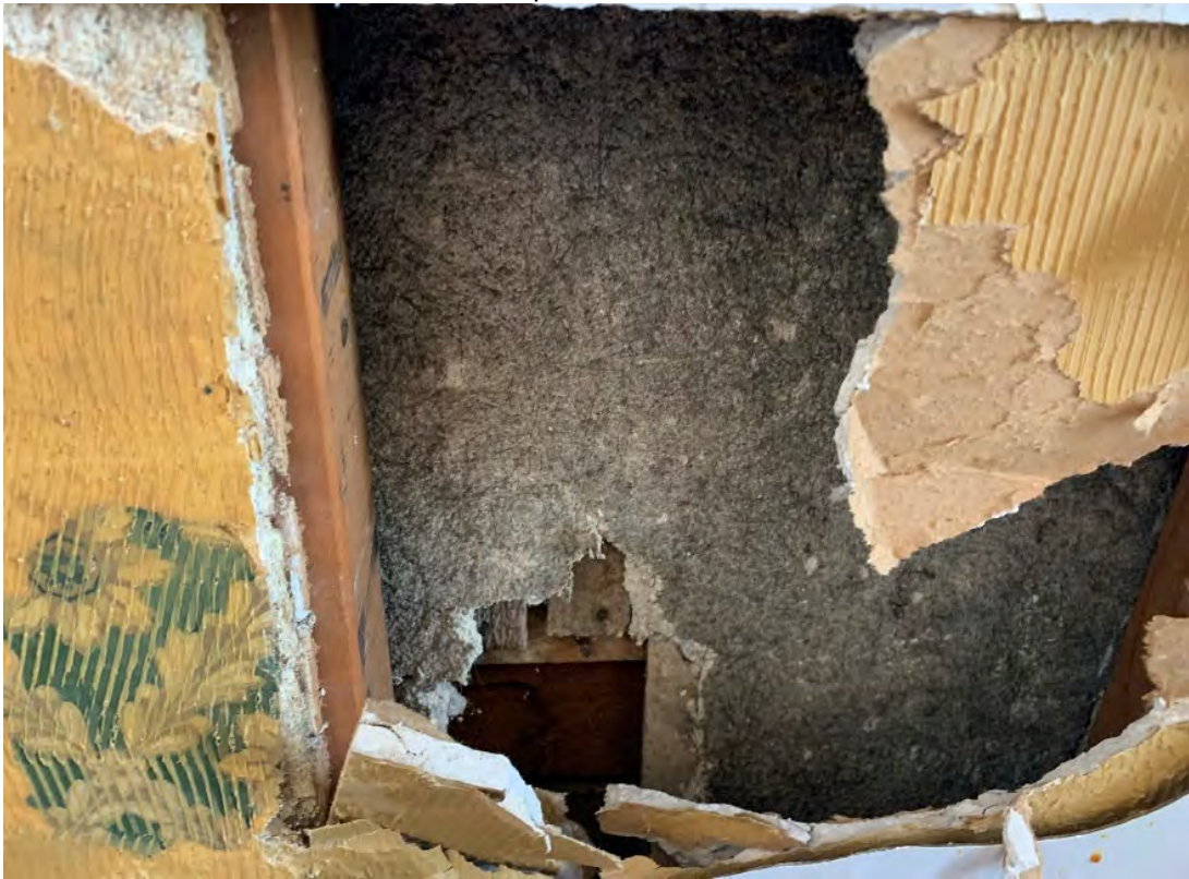
Plaster behind gypsum board wall
