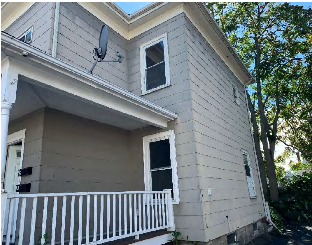
Typical Windows and doors with ACM trim Caulk
