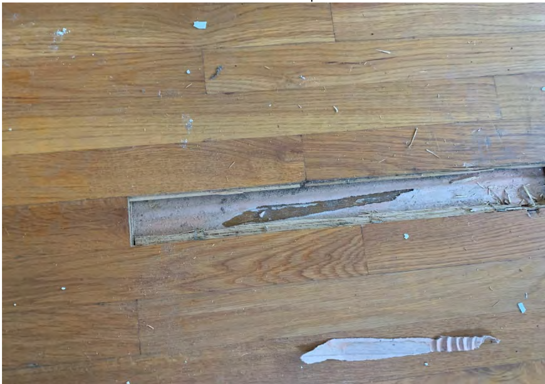
Gray paper beneath wood flooring
