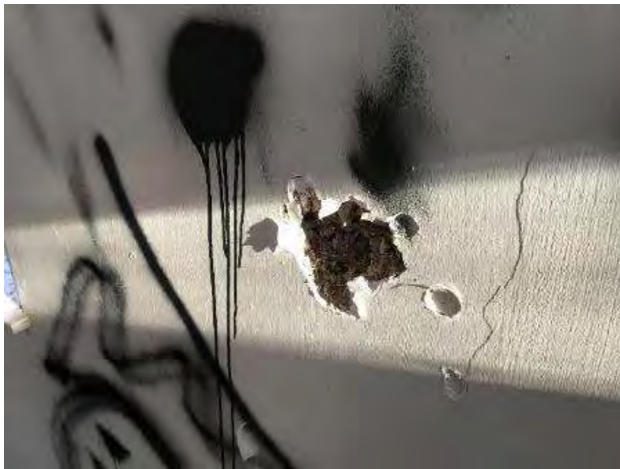
Plaster walls at the site
