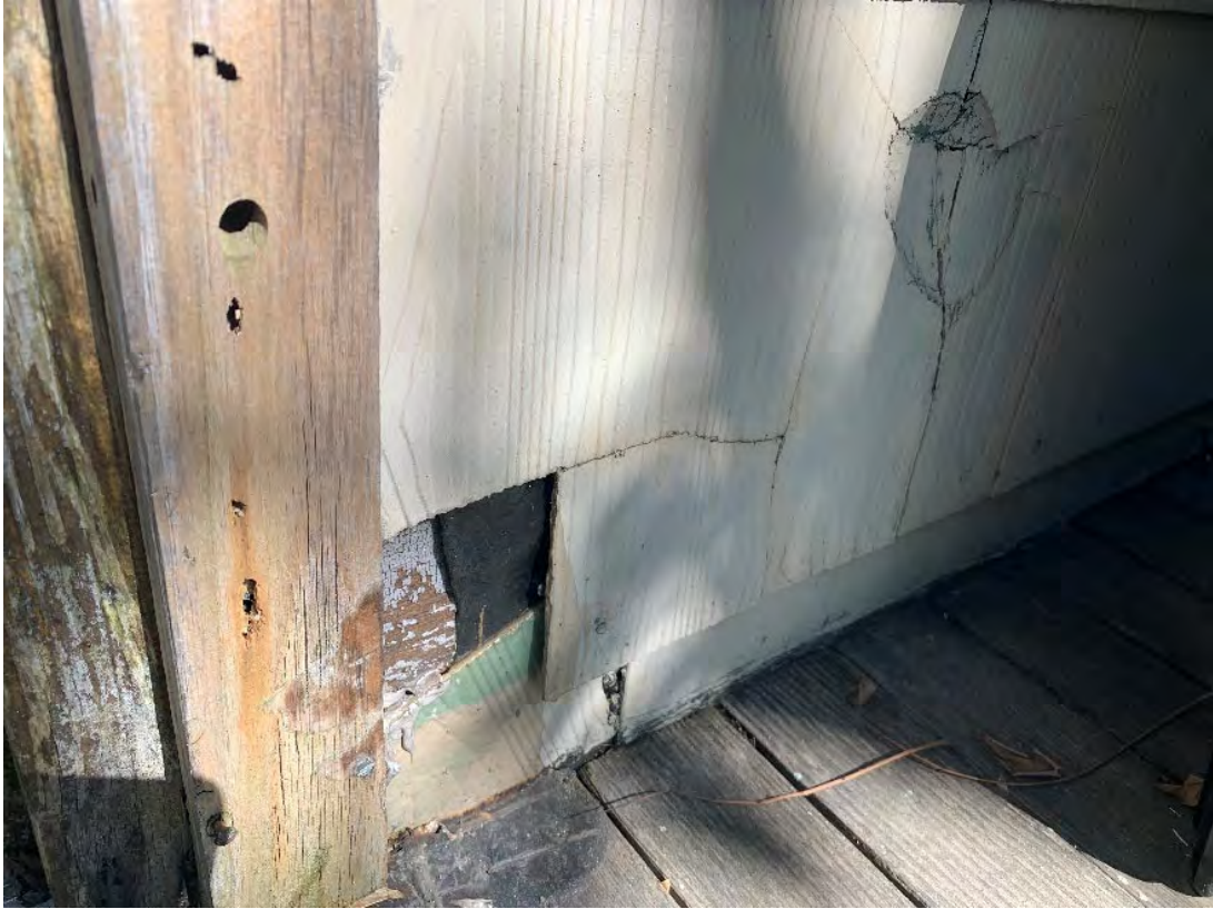
Exterior ACM cement siding
