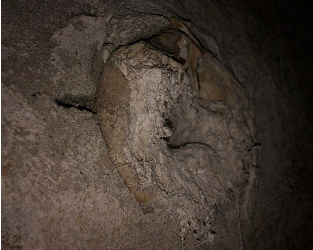
ACM Pipe Insulation
