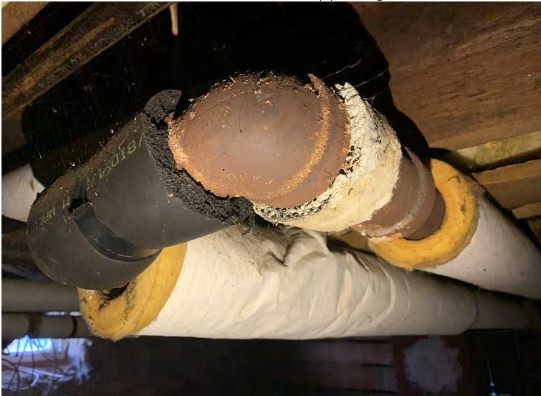
ACM pipe insulation
