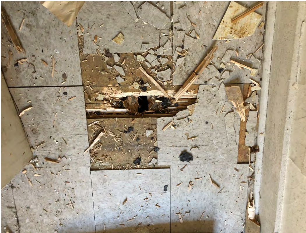
12" x 12" Tan Floor with Gray Streaks, Associated Yellow Mastic and Black Paper Under Wood Floors
