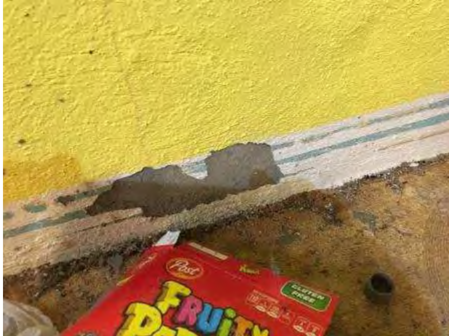
Textured paint on concrete wall
