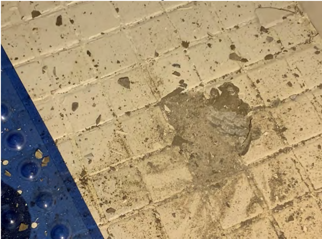
Ceramic floor tile grout and thin set
