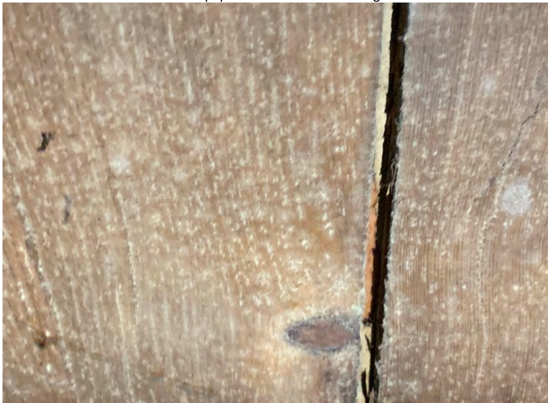
Brown paper beneath wood flooring
