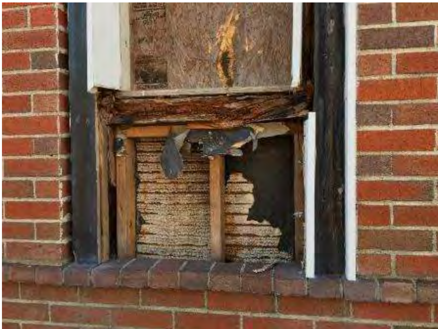
Backing sheetrock and vapor barrier behind decorative window cutouts
