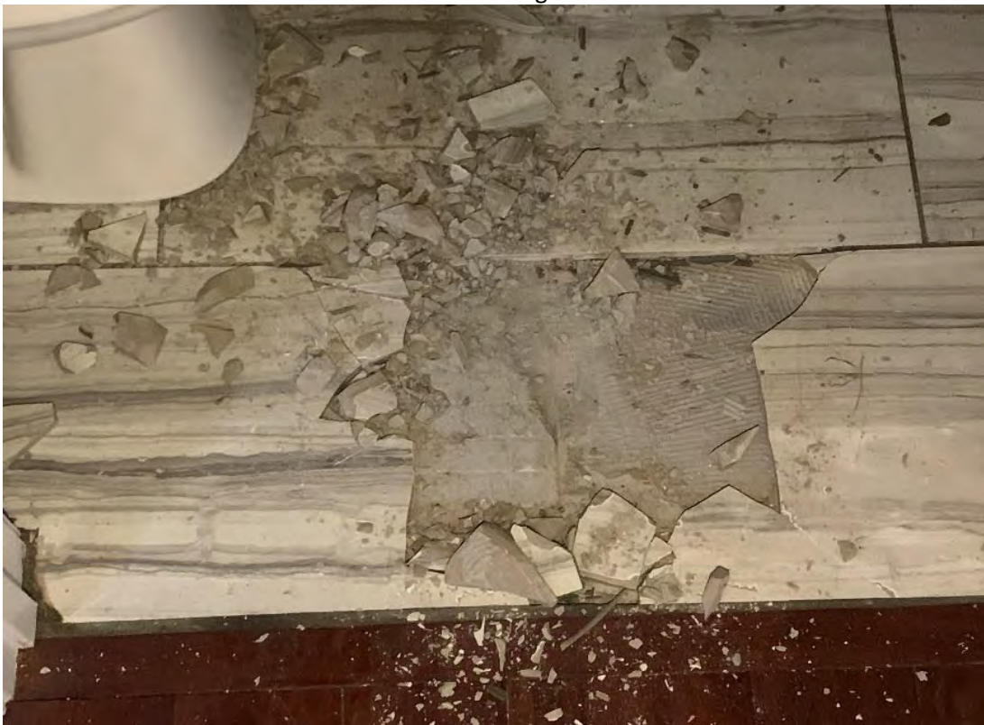
Ceramic floor tile grout and thin set
