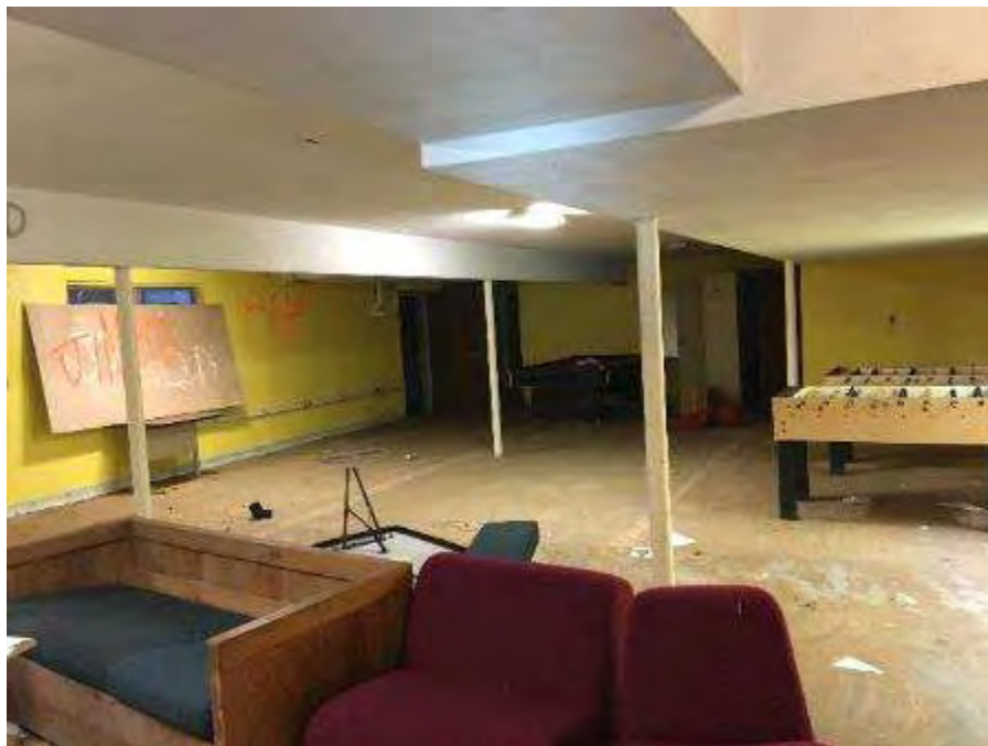
Basement rec room. Note ACM ceiling texture.
