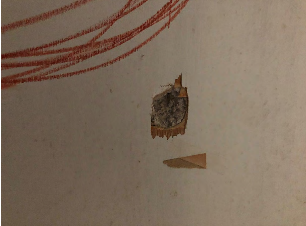
White Insulation Inside Wood Door
