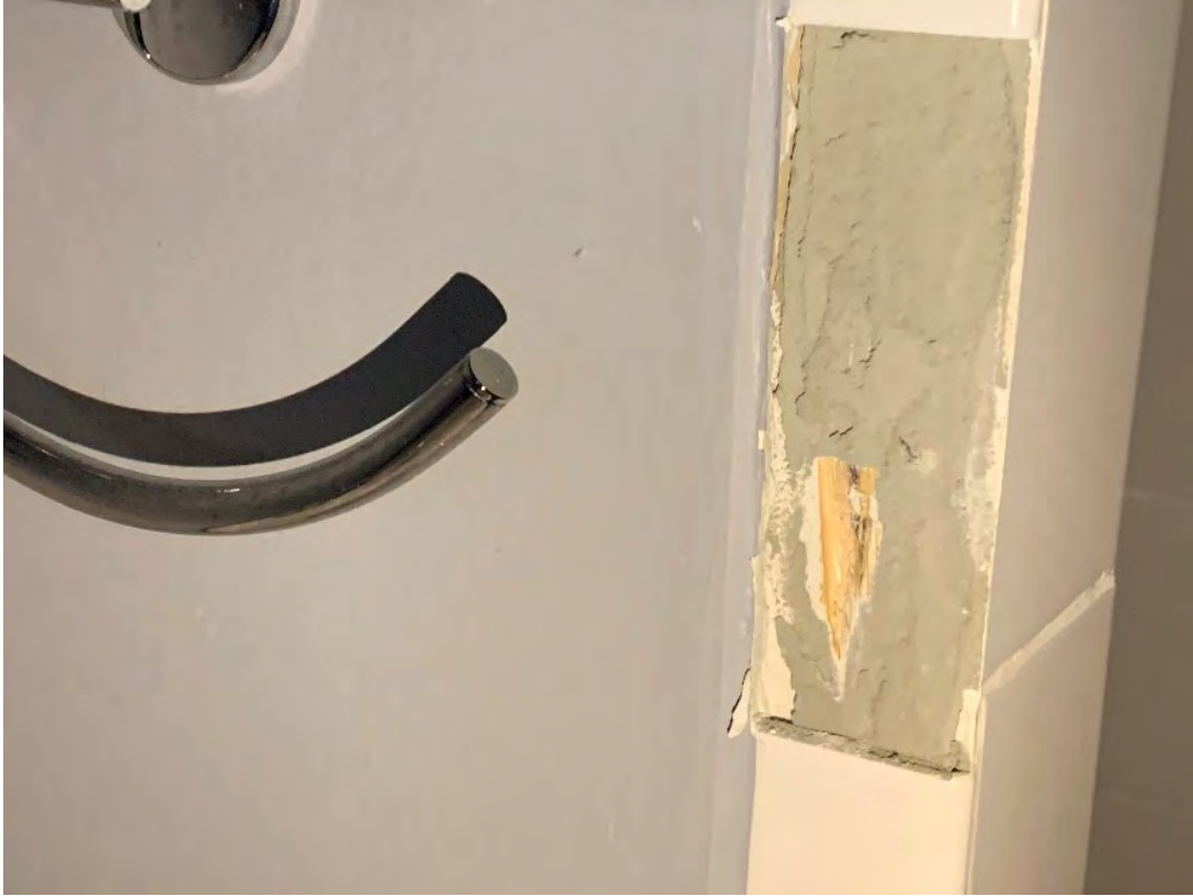
Ceramic wall tile grout and thin set
