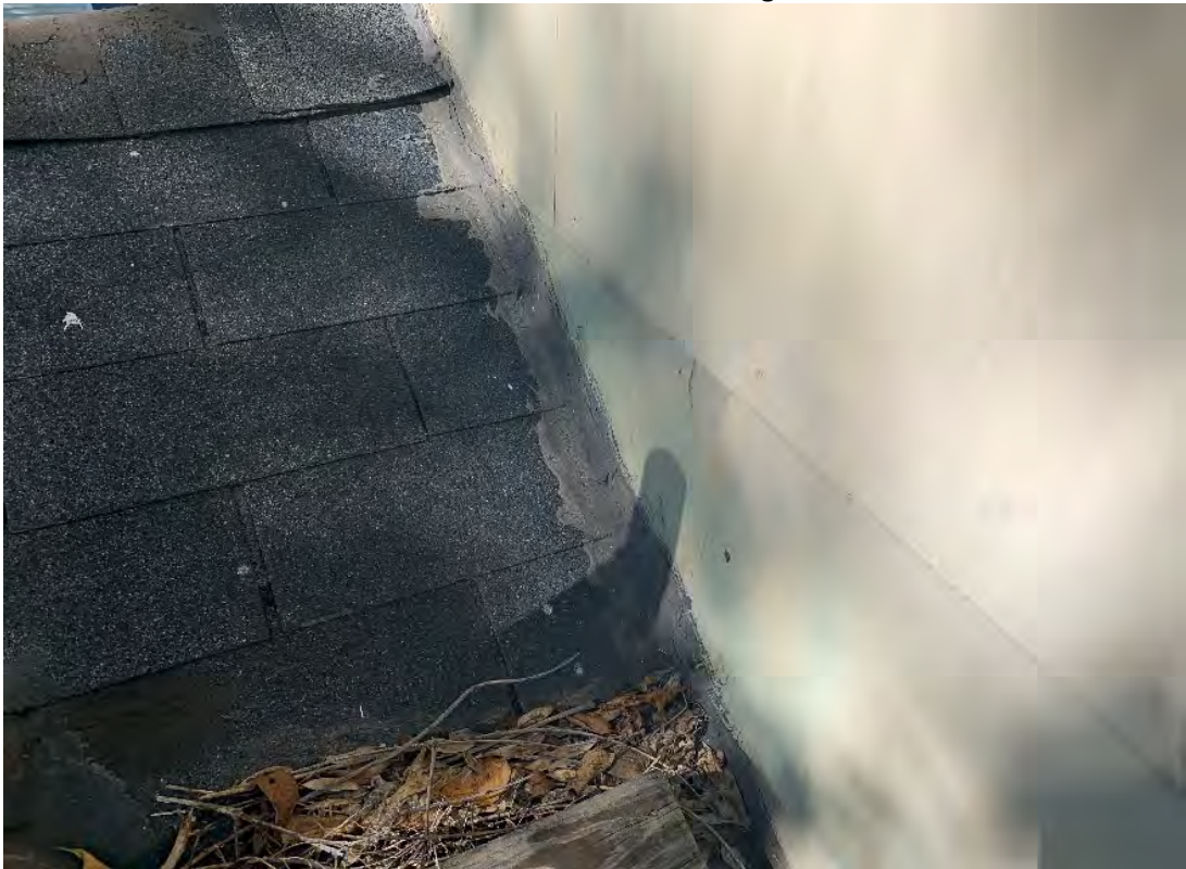
ACM black roof sealant
