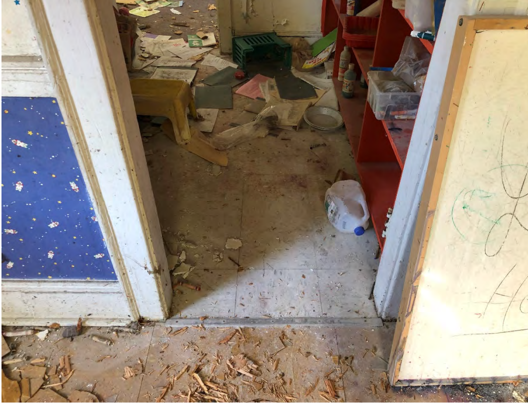
12" x 12" White Floor Tile with Gray Fleck, 12" x 12" Brown Floor Tile with Yellow Fleck and Associated Yellow Mastic
