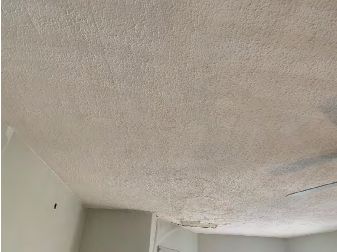
Textured plaster ceiling
