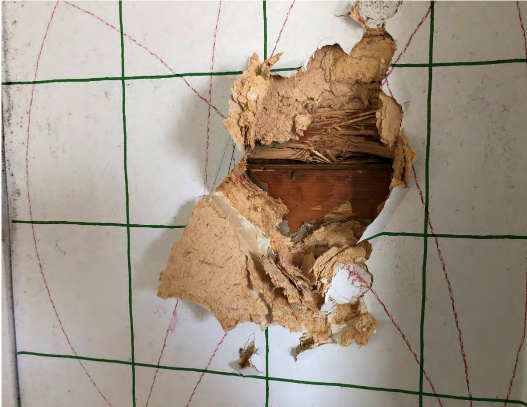
Brown Paper Behind Wood Wall
