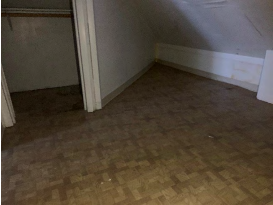
Wall base molding with adhesive
