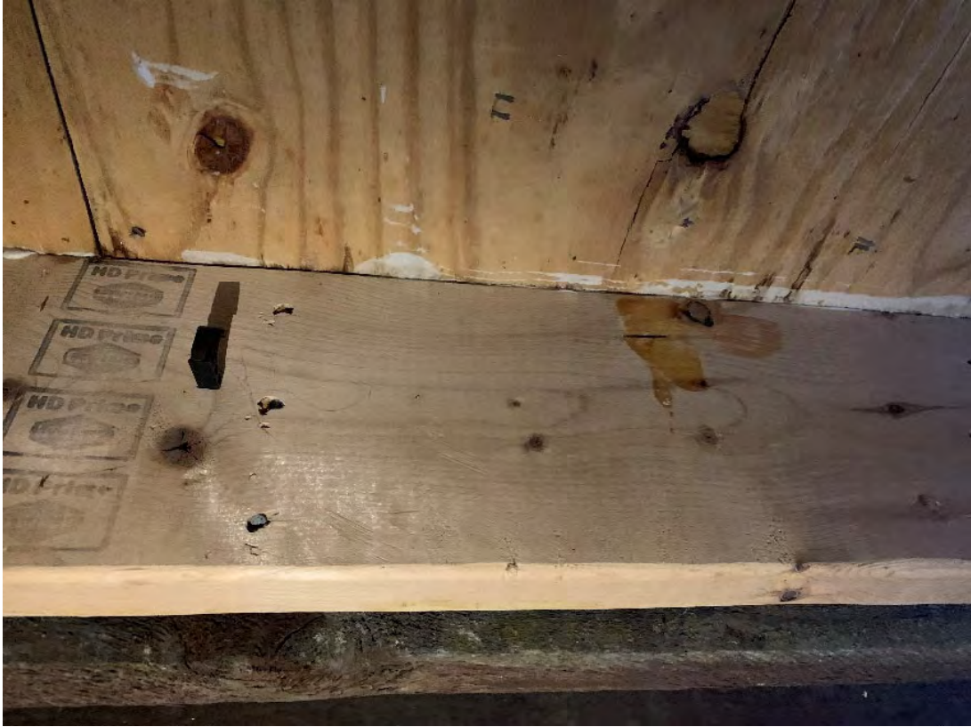
Construction adhesive on plywood flooring
