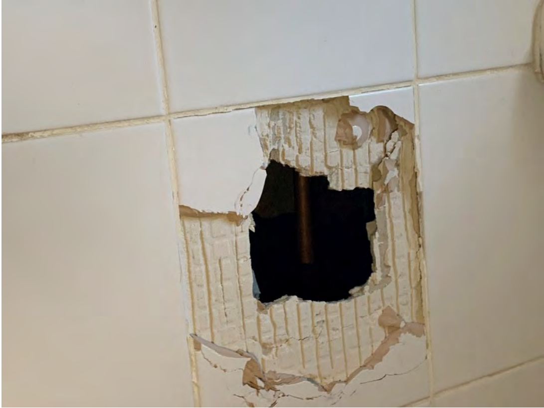
Ceramic wall tile grout and thin set
