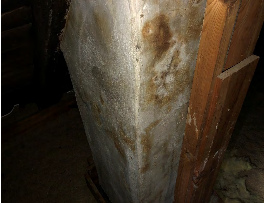
Gray Skim Coat on Chimney
