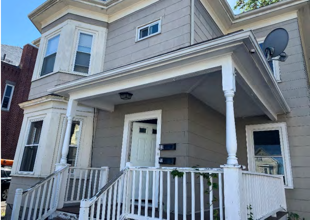
Typical Windows and doors with ACM trim Caulk
