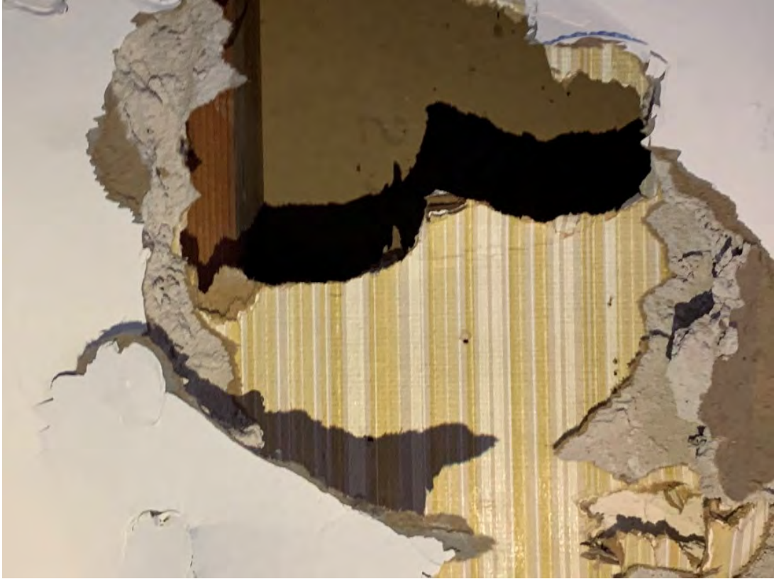
Second layer gypsum board wall
