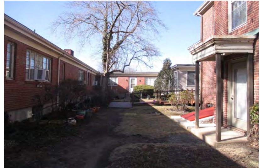
The courtyard between the Leland Home and the 1938 and 1954 additions, view north
