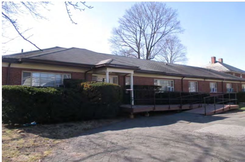
The façade of the 1952 addition, view northwest
