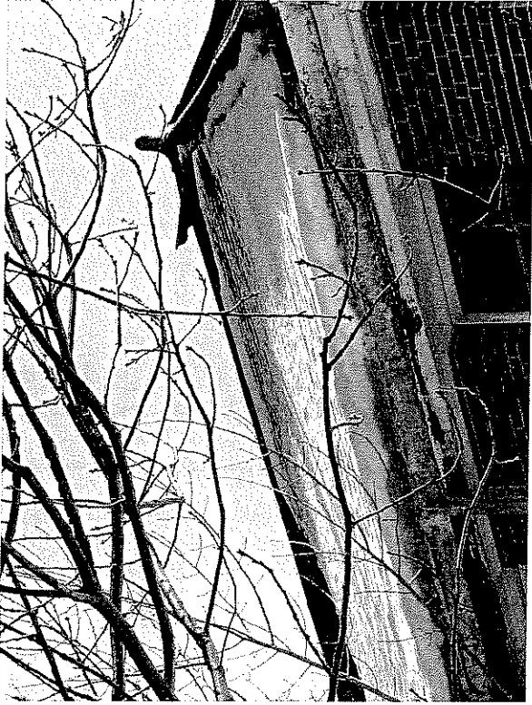
66. Detail of Roof
