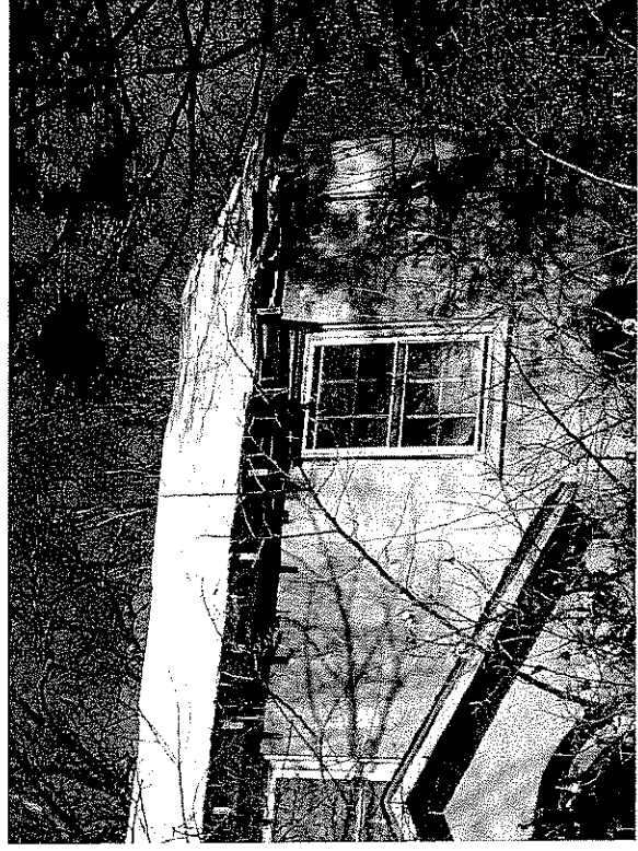
38. Detail of West Elevation
