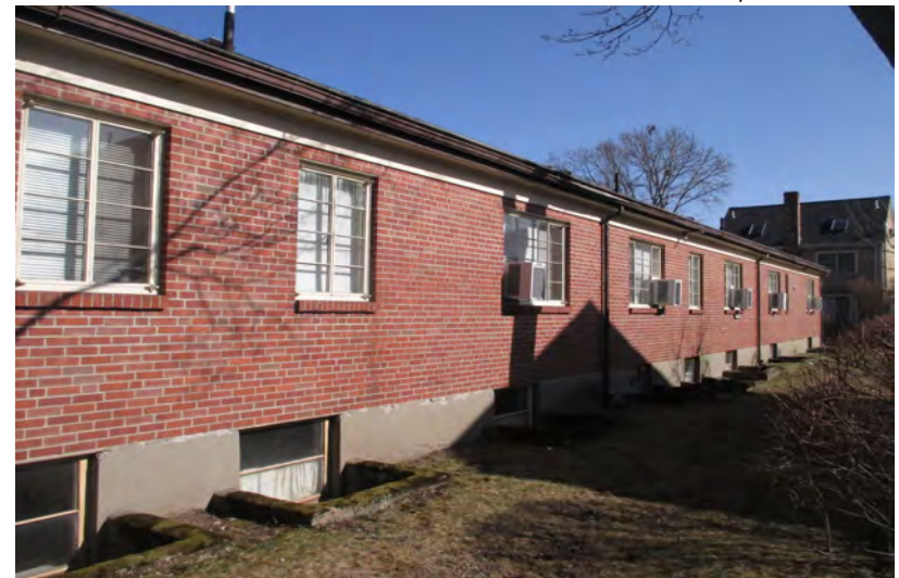
Rear (west) elevation of the 1952 addition, view southeast
