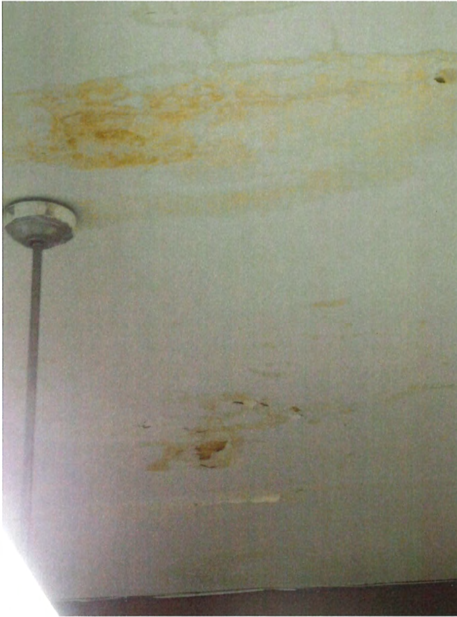
2 nd floor ceiling damage due to roof leaks (now repaired)
