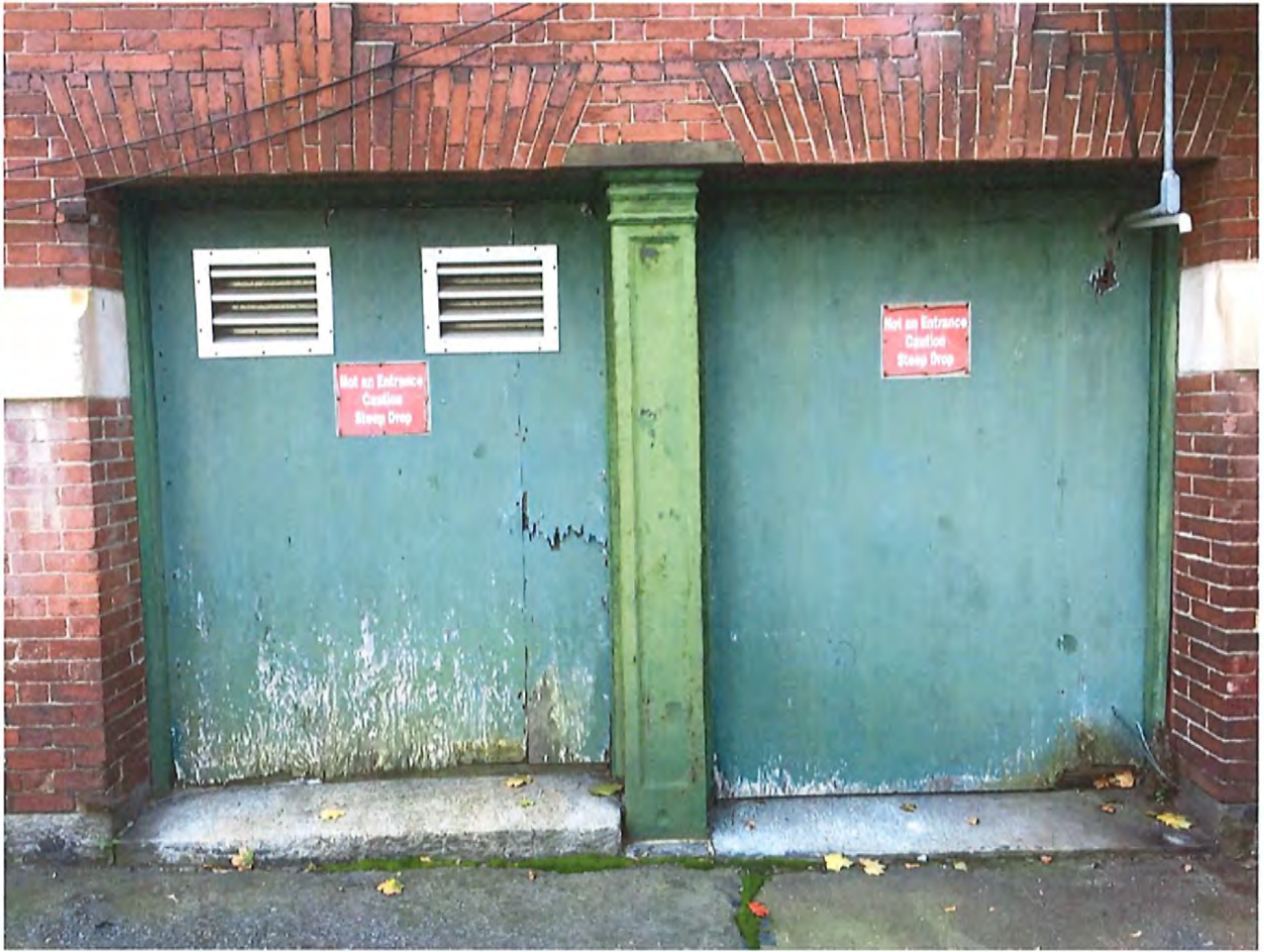
Rear wooden doors leading to boiler room. Wood is showing signs of rot.
