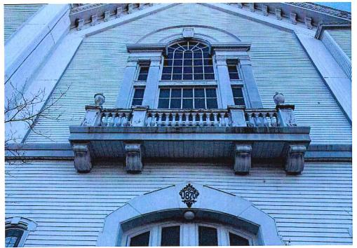
Figure 3: Front woodwork that needs restoration
