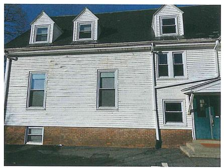
Figure 5: Warped panels from fire
