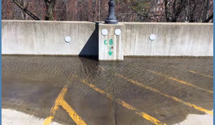
Image of stormwater puddled in a parking lot that will produce runoff containing pollutants absorbed from the surface of the asphalt.
