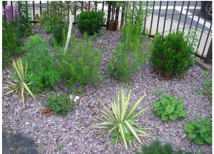
Example of a small bioretention area called a rain garden. Stormwater flows from the parking lot into the garden where vegetation absorbs some of the storm-water and excess nutrients in it.
