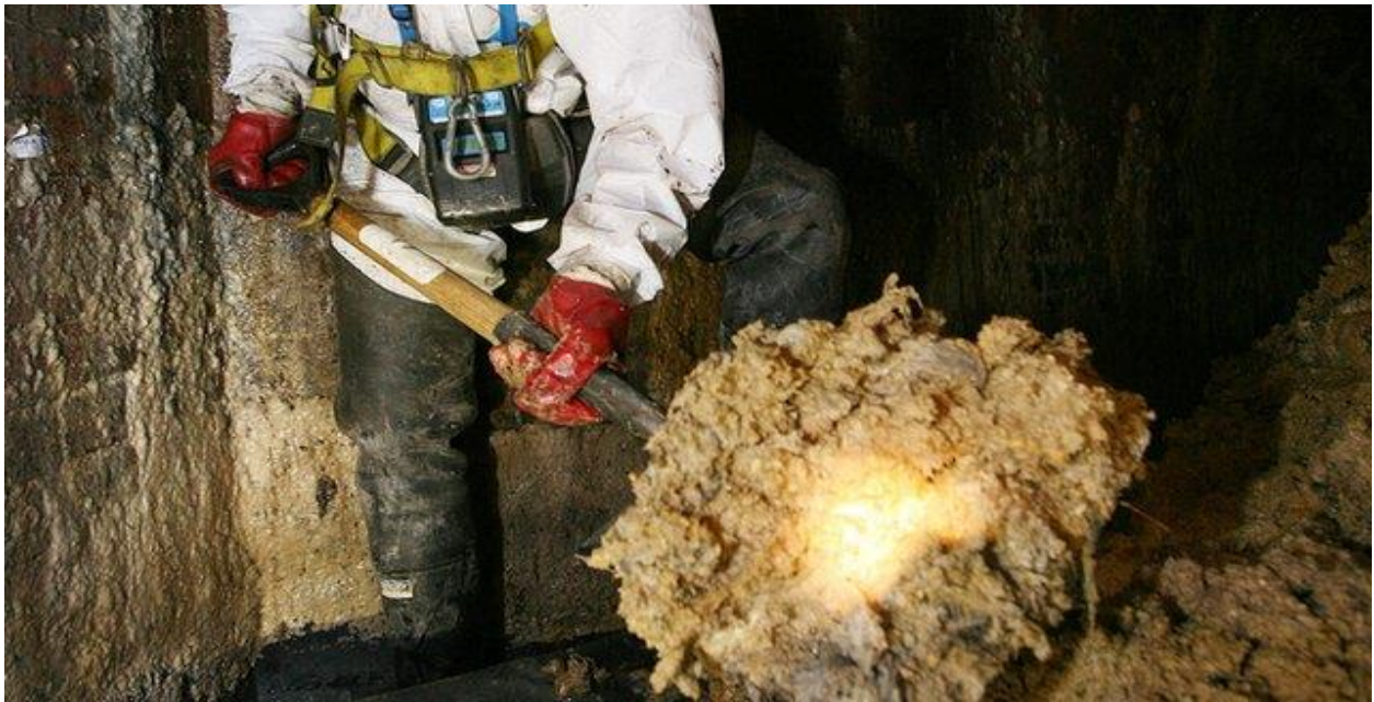
FOG in City Sewers Can Build Up Causing Significant Obstructions in Pipes & Manholes
