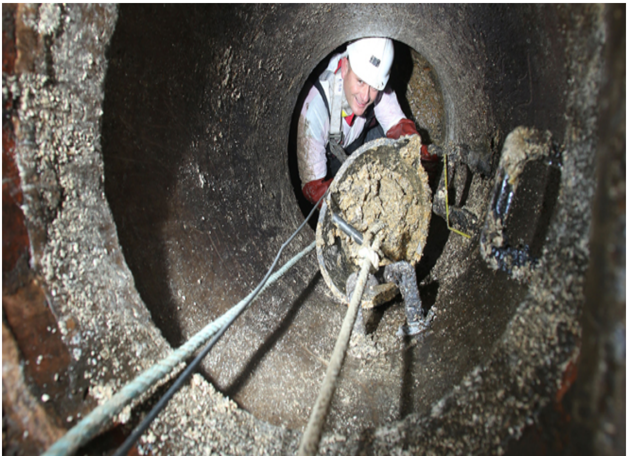
Damage to Manholes and Sewer Lined Caused by FOG Build-Up
