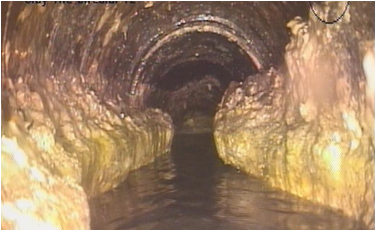
FOG Buildup in Sewer Pipe
