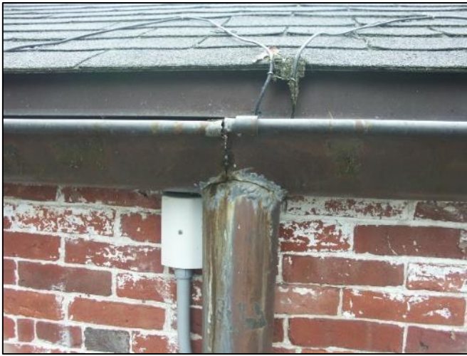
Typical downspout / gutter on north elevation of c. 1804 greenhouse.
