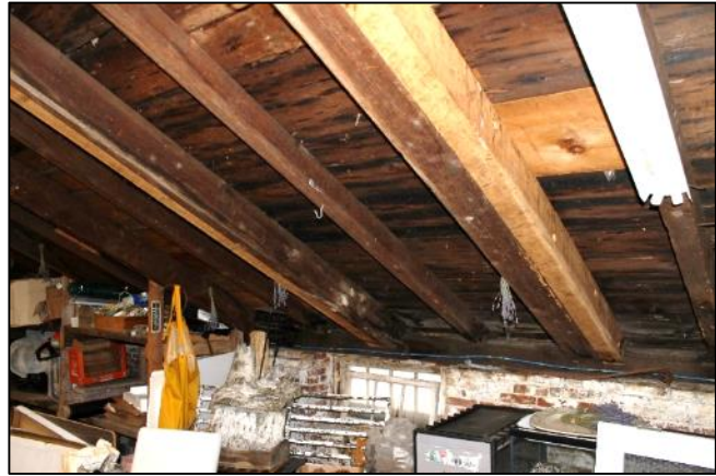
Alternating principle and common rafters in c. 1804 greenhouse. Two principle rafters with “sisters” shown here illustrate 1997 repair work
