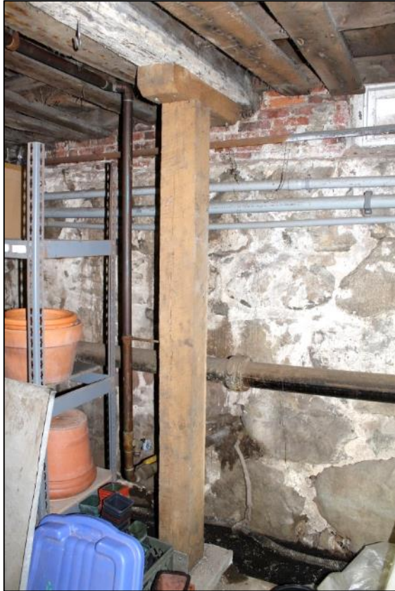
Framing structural repair (c. 1997) in c. 1804 greenhouse basement.
