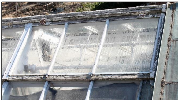
Typical conditions of roof vent sash and ridge assembly showing cracks, checks, old screw holes and paint failure.
