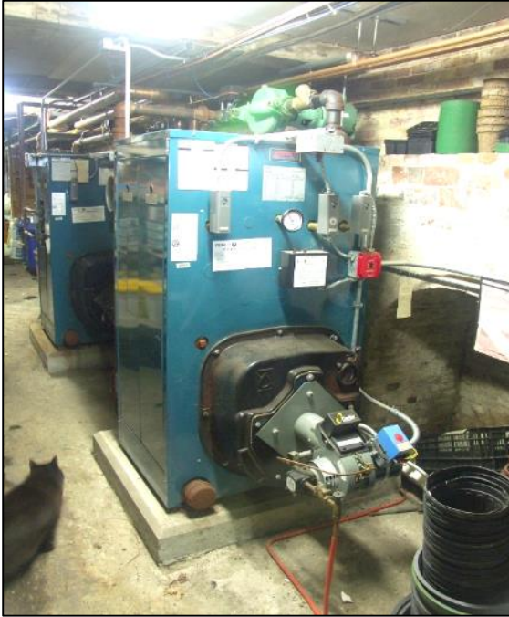
Greenhouse boilers Burnham low pressure V904A.
