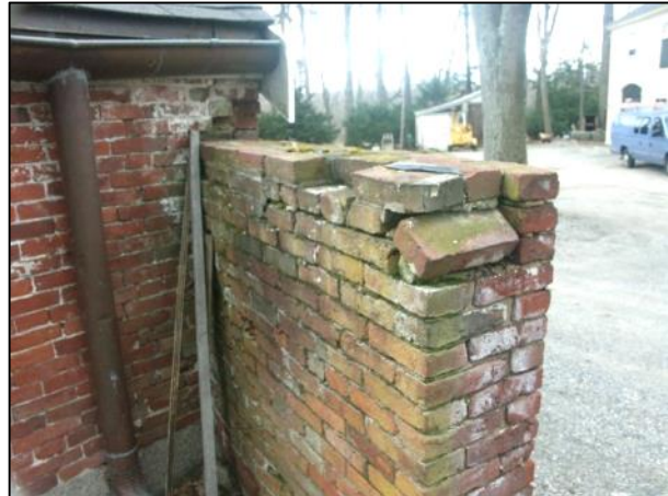
Loss bricks at entry wall.
