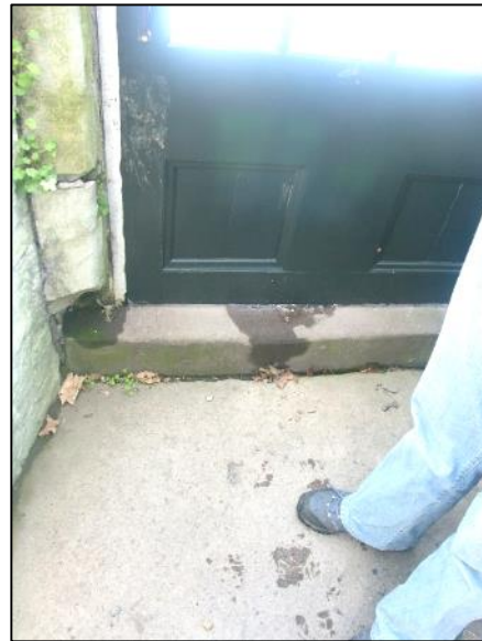
Water leaking back into the entry from ice dams at the c. 1804 greenhouse.
