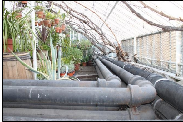
Supply and return runs visible in the "Grape House."
