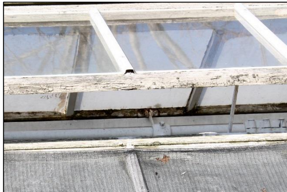
Typical conditions of interior of roof vent sash showing deterioration at bottom rail
