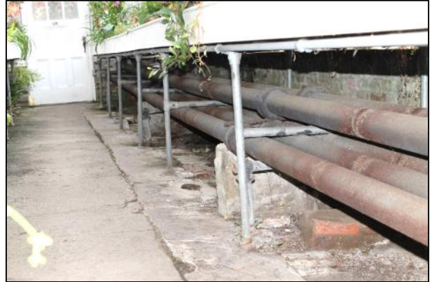
Typical 5" cast iron heating pipes.
