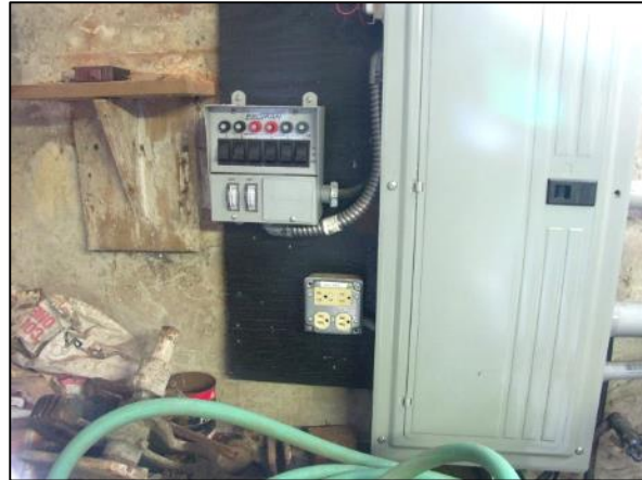
Generator transfer switch next to panel at west end of c. 1804 basement.
