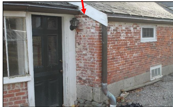
Deteriorated mortar on the north elevation of the "Grape House."
