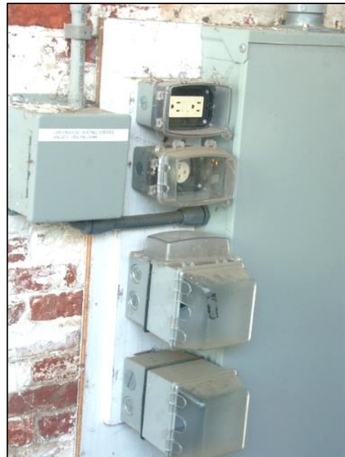
Dedicated circuits for auxiliary heaters (2) 50 amp, 240v, (1) 20 amp, 240v.
