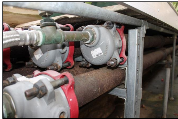
Example of repairs to existing piping in the "Camellia House."
