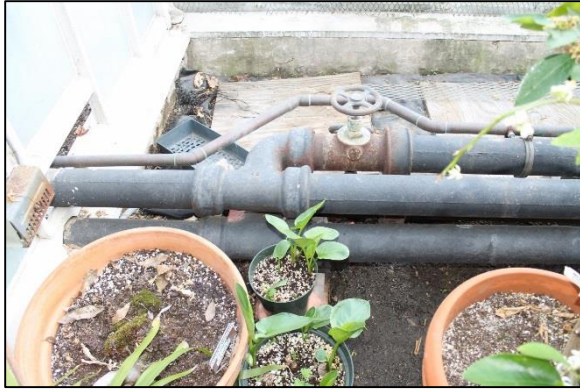
Example of 5" cast iron runs with gate valves for control in the "Grape House"
