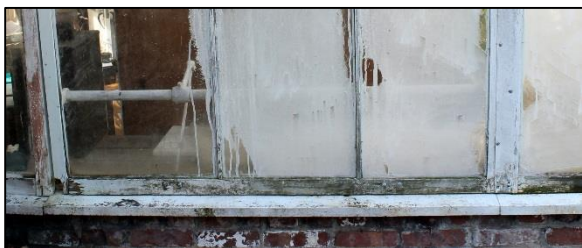
Sample conditions of side wall sash showing wood deterioration and paint failure
