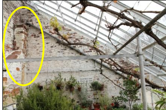
Remnants of chimneys in the c. 1804 greenhouse (top: west; bottom: east).
