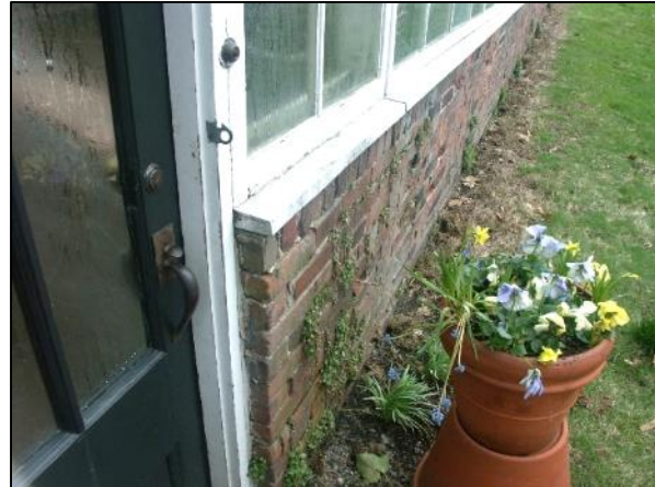
Building impact due to drainage at entry of c. 1804 greenhouse.
