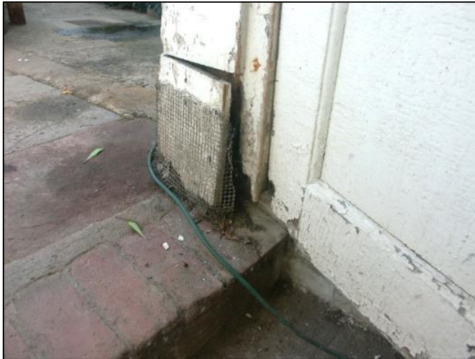
Door to basement of c. 1804 greenhouse showing rot in trim.
