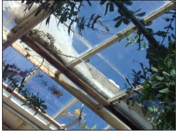
Cracked glass in c. 1804 greenhouse – results in leak over walkway impacting visitors.
