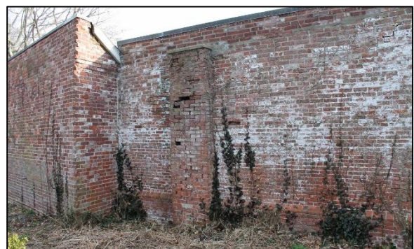
Deteriorated mortar on the north elevation of the "Orchid House."
