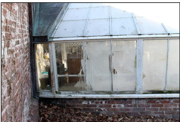
Sample conditions of side wall sash showing wood deterioration and paint failure
