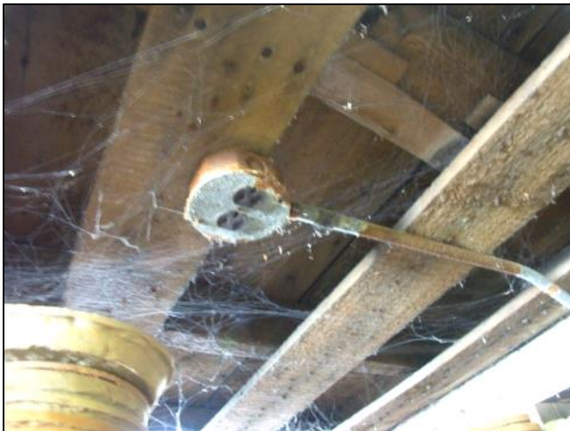
Rusty outlet and conduit in c. 1804 storage area.
