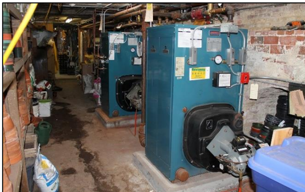
Existing hydronic boiler setup.
