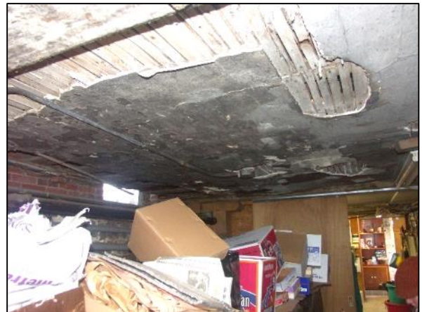
Plaster failure in the boiler room ceiling of the c. 1804 greenhouse.
