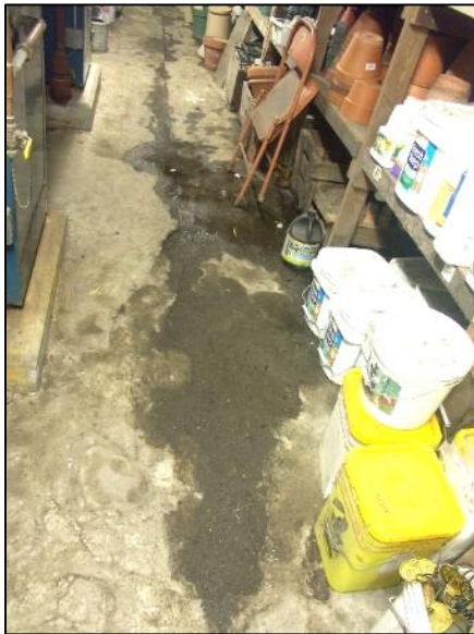
Wet floor near boilers, 24 hours after heavy rains.
