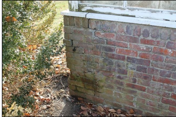
The east end of the "Grape House" requires significant masonry repairs where the corner and peak are losing structural integrity.
