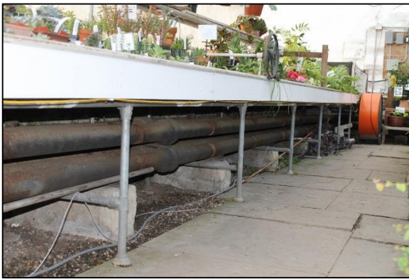
Example of 5" cast iron runs in the "Sales House."
