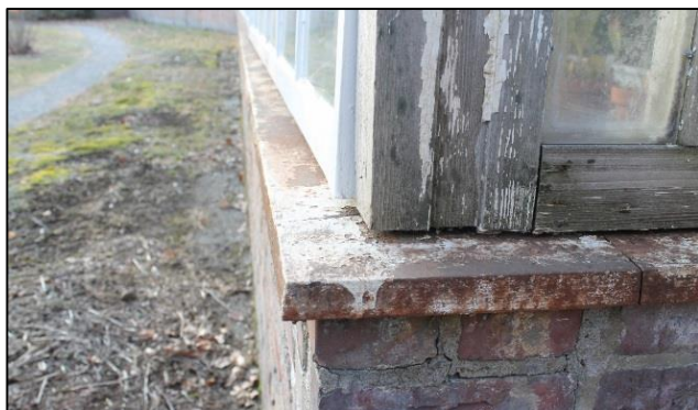
Typical conditions of metal sills/wall caps.
