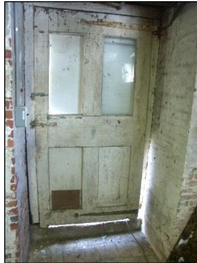
Door to basement of c. 1804 greenhouse with lower strap hinge and pintle missing.
