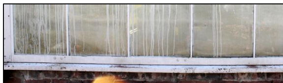
Typical conditions of metal sills / wall caps; note wear points indicating binding of sash hastening deterioration of operable sash
