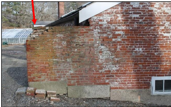
Masonry damage to the west end of the "Grape House."
